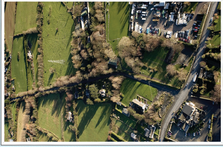
View looking south along the Glenamuck Road showing the Golden Ball junction to the bottom left/centre and High Voltage ESB services to the top centre. Wayside Celtic sports ground is to be relocated to the top right.
