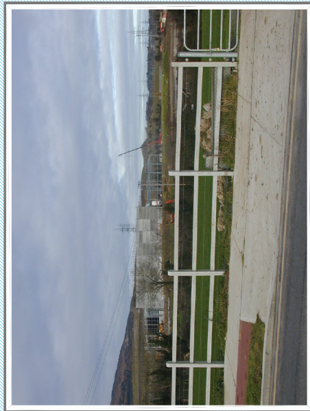
View looking west from the Glenamuck Road showing Park Developments under construction and High Voltage ESB lines leading to Carrickmines Powerstation.
