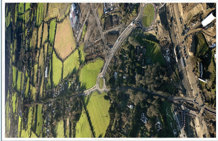
View looking south along the Glenamuck Road showing the Carrickmines Interchange Southern Roundabout to the middle centre. The South Eastern Motorway is under construction to the bottom of the photograph.
