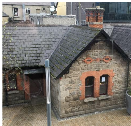
Photo 5.2: Red Brick features around door, windows, chimney and over window detailing, Pembroke Cottages, Ballinteer Road
