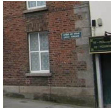
Photo 5.4: Granite dressing on red brick building, Eagle Terrace
