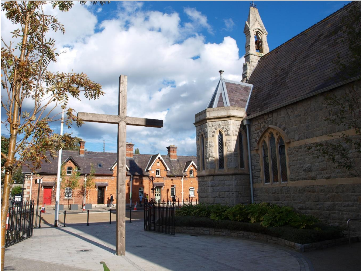
Photo 5.13: View of Holy Cross side elevation towards Pembroke Cottages.
