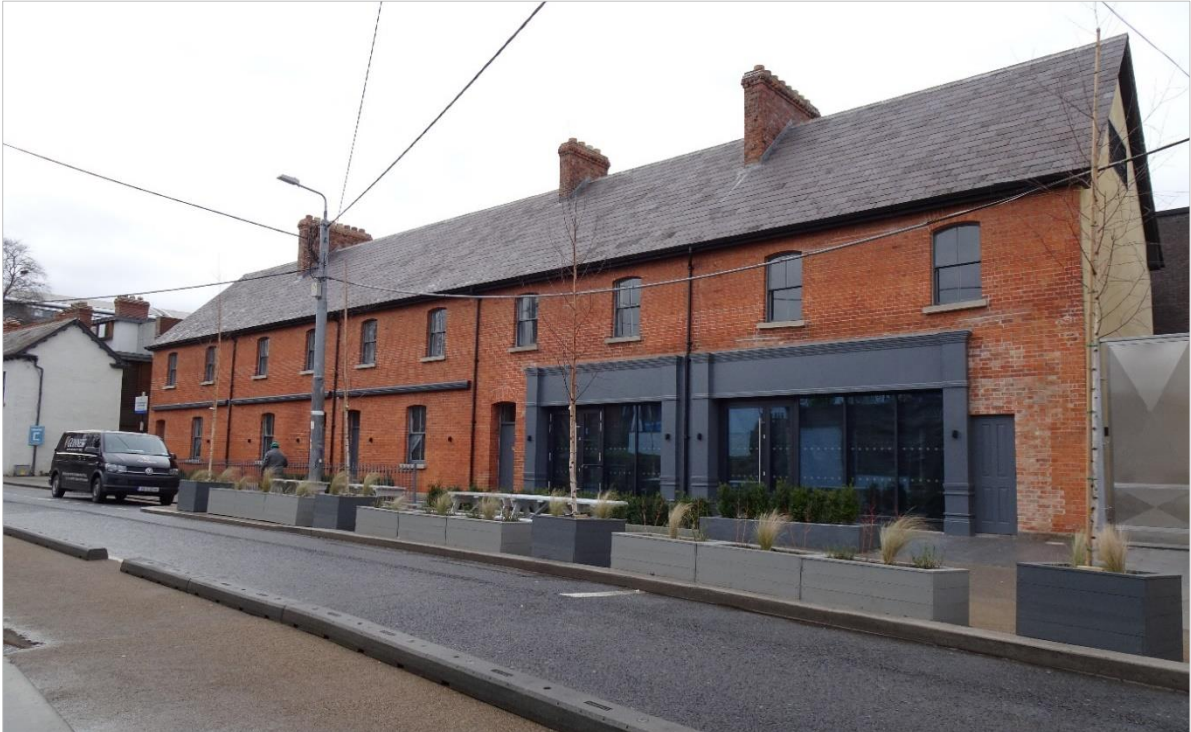
Photo 5.17: Ashgrove Terrace post refurbishment (January 2021)
