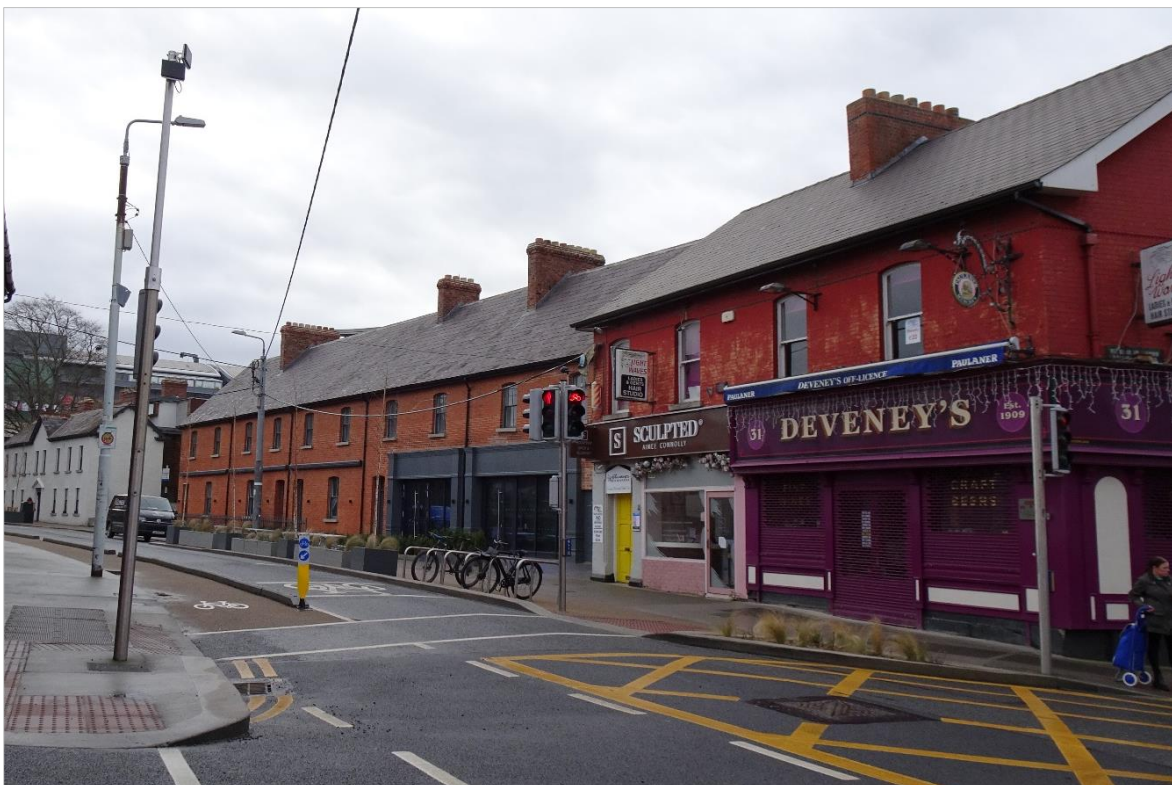
Photo 5.15: Deveney's Public House (now off-licence) with Ashgrove Terrace and the Mill House in background
