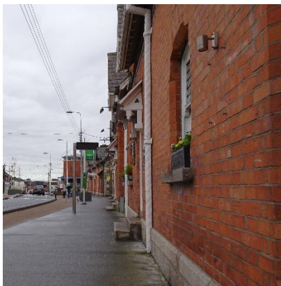
Photo 5.1: Red brick in use at Pembroke Cottages, Main Street
