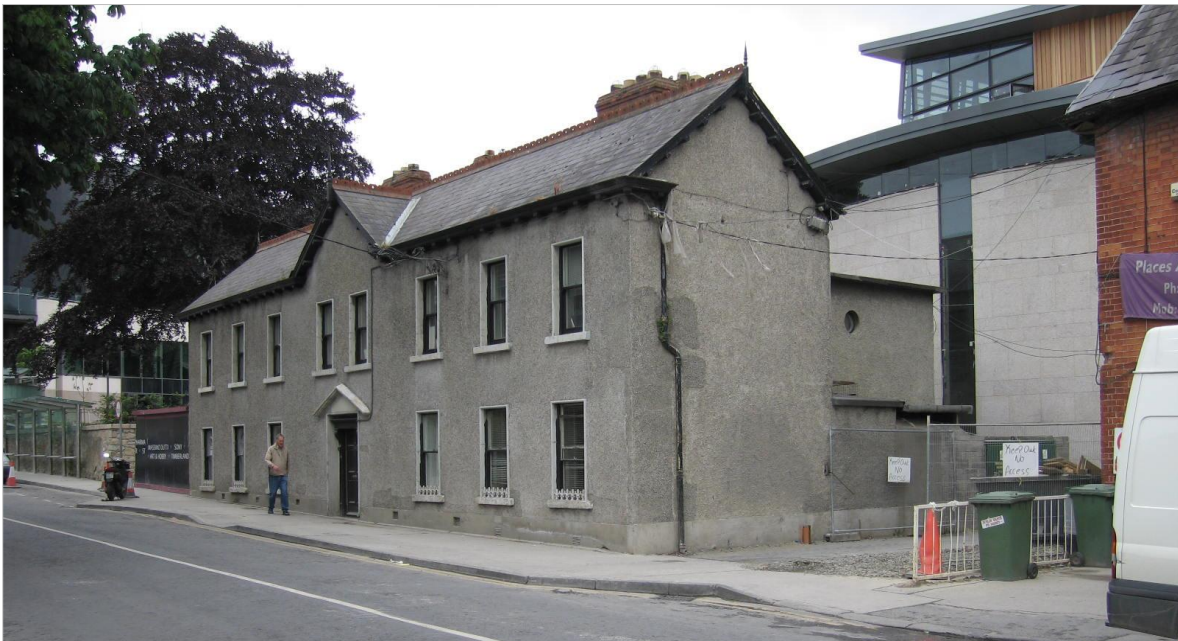
Photo 5.19: The Mill House, Sandyford Road
