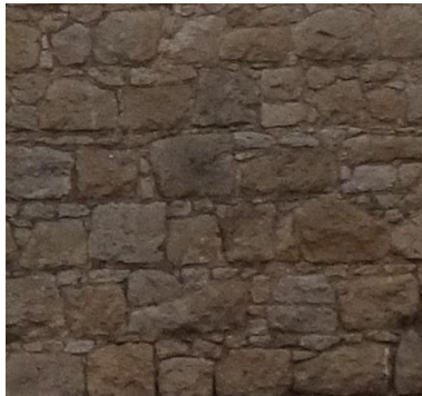
Photo 5.3: Granite rubble finish, Pembroke Cottages, Ballinteer Road
