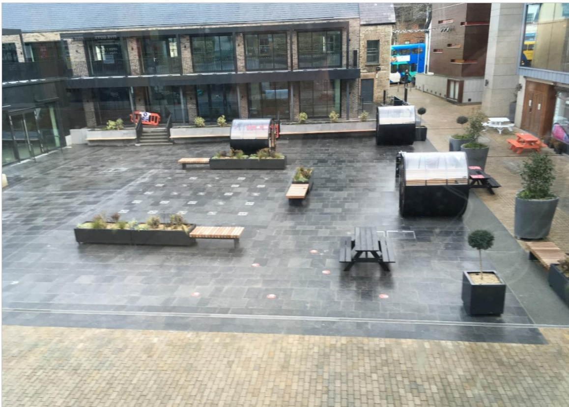
Photo 5.27: Recently completed public space (referred to as Pembroke Square) to the rear of Ashgrove Terrace.
