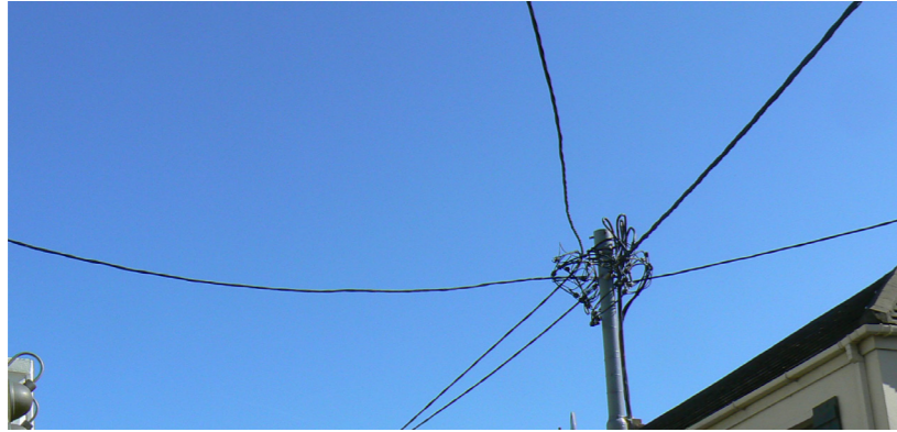
Photo 90: Overhead Power Lines
