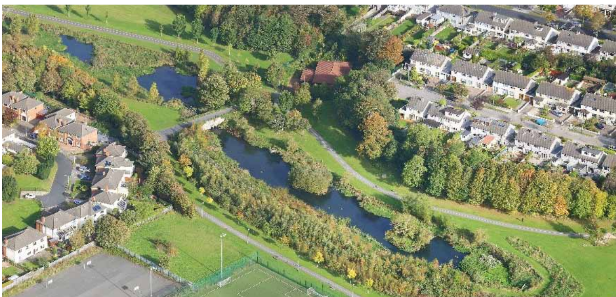
Kilbogget Park - site of proposed Flood Storage Area
