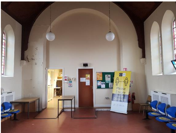
Photo 9: Nave looking East
