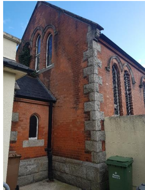
Photo 4: Entrance Porch & Western Gable
