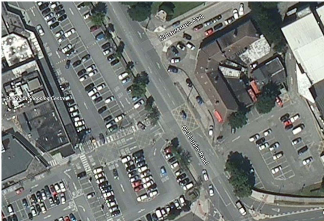
Figure 5.5 Existing Junction Layout (Satellite)
