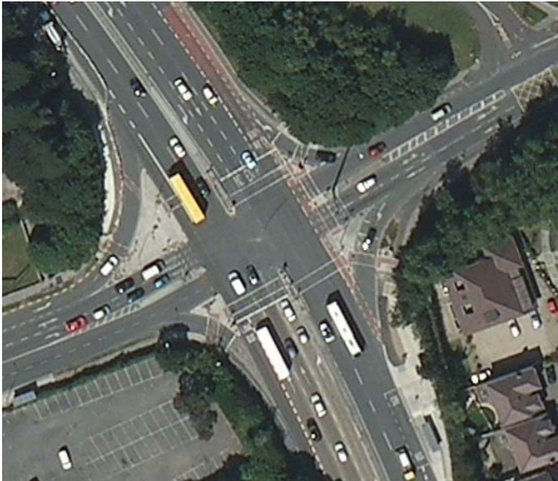
Figure 5.11: Existing Junction Layout (Satellite)
