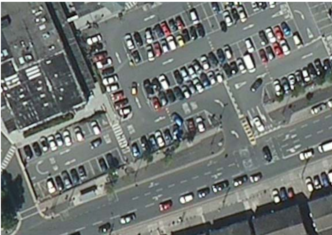
Figure 5.3: Existing Junction Layout (Satellite)
