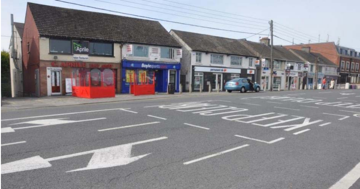
Figure 2.3: Wide carriageway width on Lower Kilmacud Road adjacent Shopping Centre
