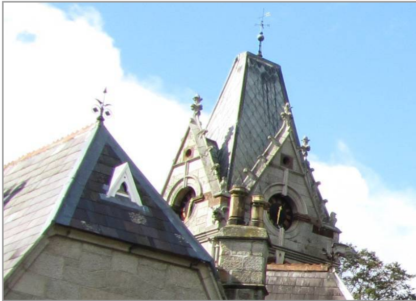
Plate 4: Decorative vent on hipped gable roof and metal decoration on the roof apices
