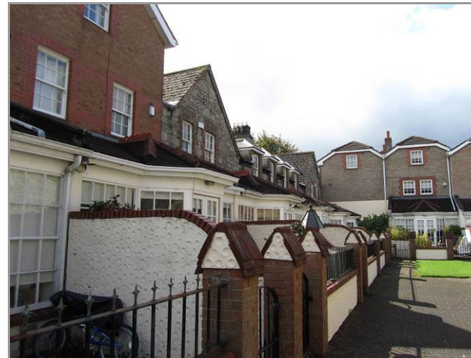
Plate 18: View of modern rear extensions to the central space
