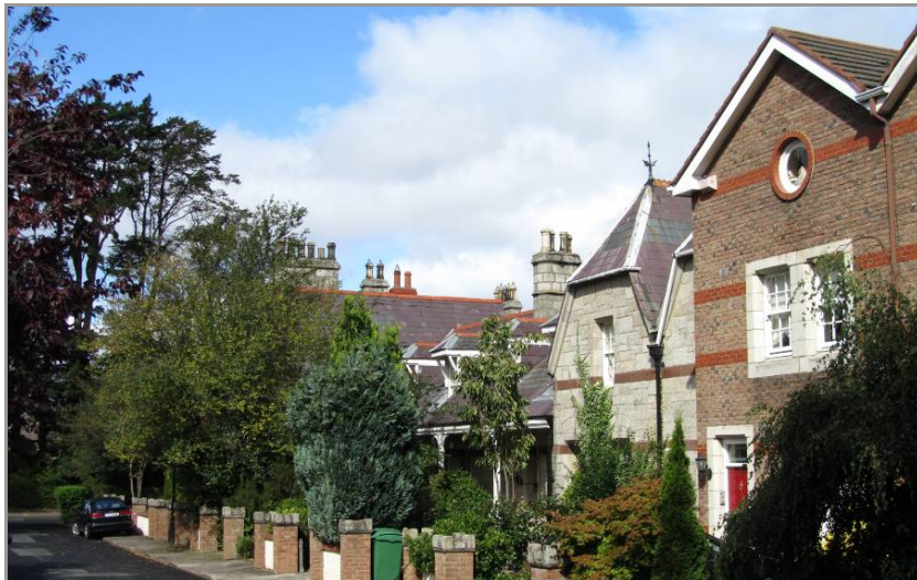
View 3: The south elevation
