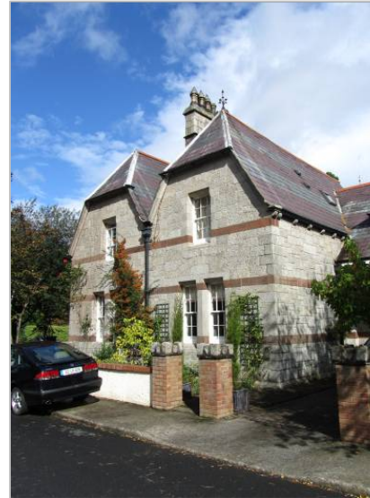
Plates 1 and 2: Banded slates and dormers with slate
