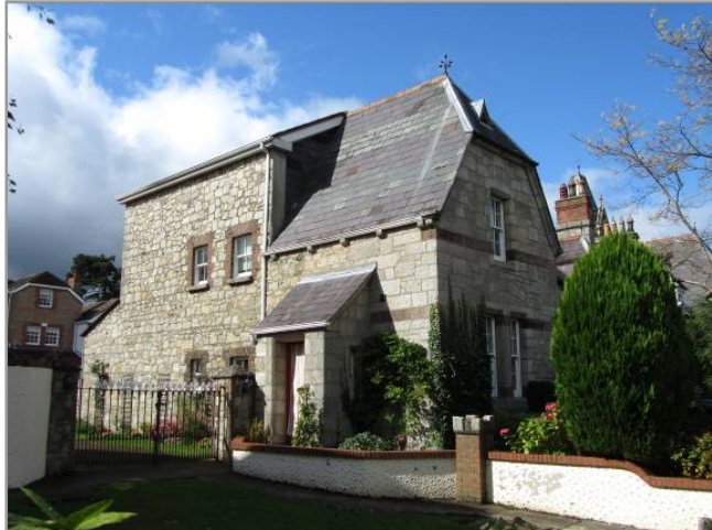
Plate 20: Inappropriate addition of large volumes to the rear of historic houses
