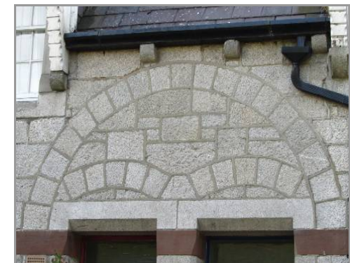
Plates 7, 8 and 9: Stone pattern and decorative arches to the elevations and use of brick
