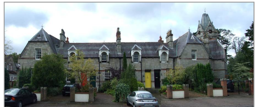
View 5: The north elevation
