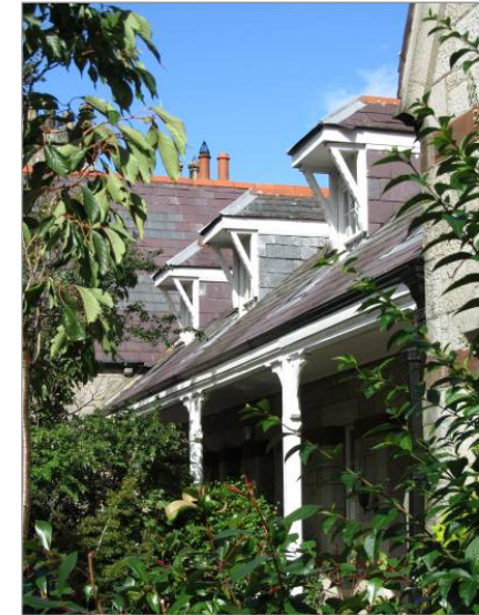
Plates 1 and 2: Banded slates and dormers with slate
