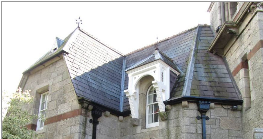
Plate 3: Roof slates, clay ridges and corner flashings
