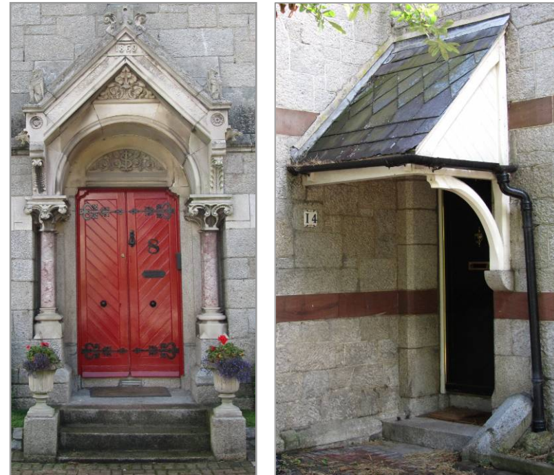
Plates 16 +17: Double doors to the tower with decorative stone surround and external canopy
