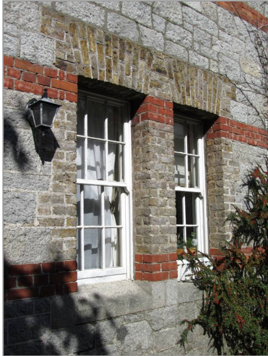
Plate 19: Stone, brick and painted timber windows
