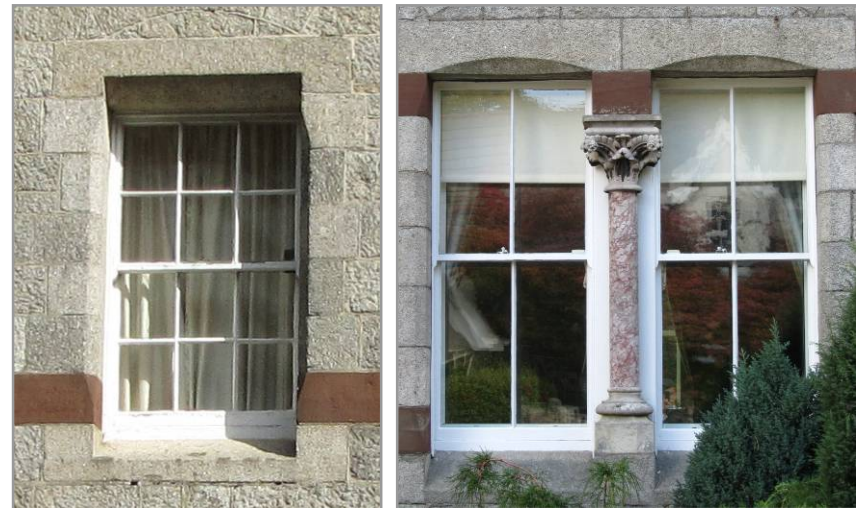
Plates 12+13: Examples of six-over-six and two-over-two timber sashes with central decorative column
