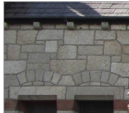
Plates 7, 8 and 9: Stone pattern and decorative arches to the elevations and use of brick
