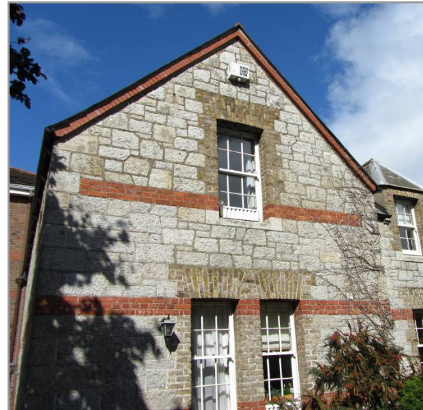
Plates 7, 8 and 9: Stone pattern and decorative arches to the elevations and use of brick
