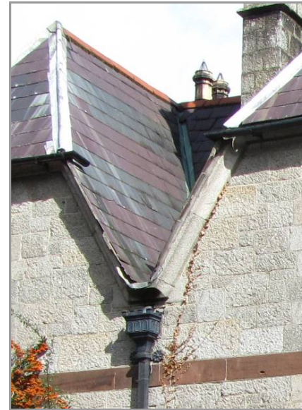
Plate 5: Return gutters and gutters resting on stone corbels
