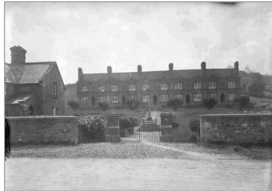
Fig 4: Almshouses in Castleblayney built c. 1879 (courtesy of the National Library of Ireland).
