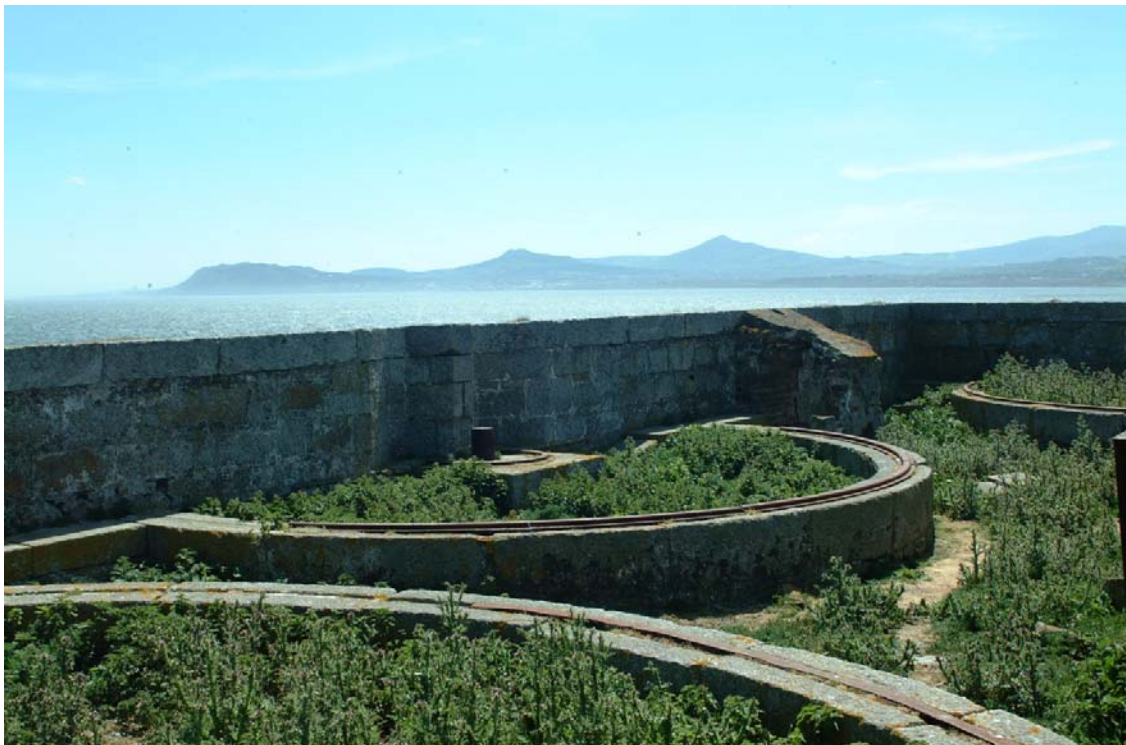
Above: Detail showing the semi-circular emplacements which housed the guns, with a shot furnace attached to the inside of the battery wall..
