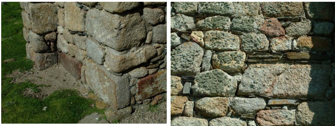
Above: Granite is the predominant stone type found at St Begnet's Church, seen here at the west door and adjacent antae. Stones at the base of the wall are sometimes 'edge-bedded' in a pseudo-cyclopean masonry style. 49
