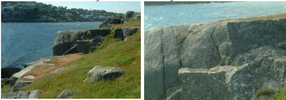
Above: Contemporary view of the quarry adjacent to the Martello tower showing a levelled quarry bed (left) retaining tool marks and blast holes in the rock face (right).
