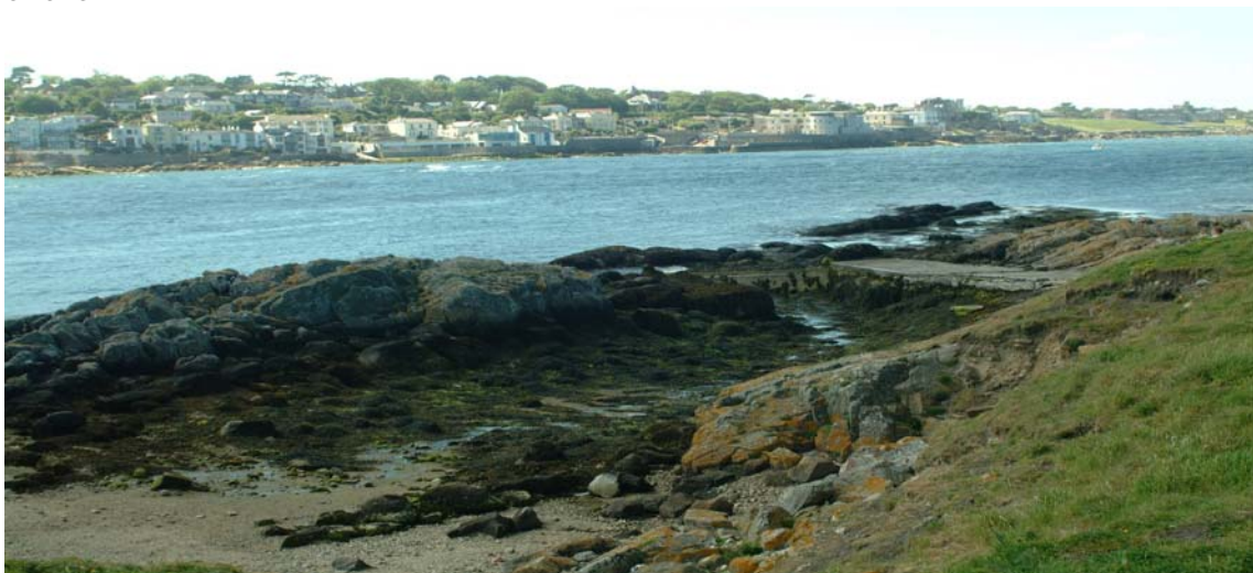
Above: General view of the boat harbour showing the quarried vertical faces of the harbour, and massive upright granite orthostats used to line the east side of the harbour.
