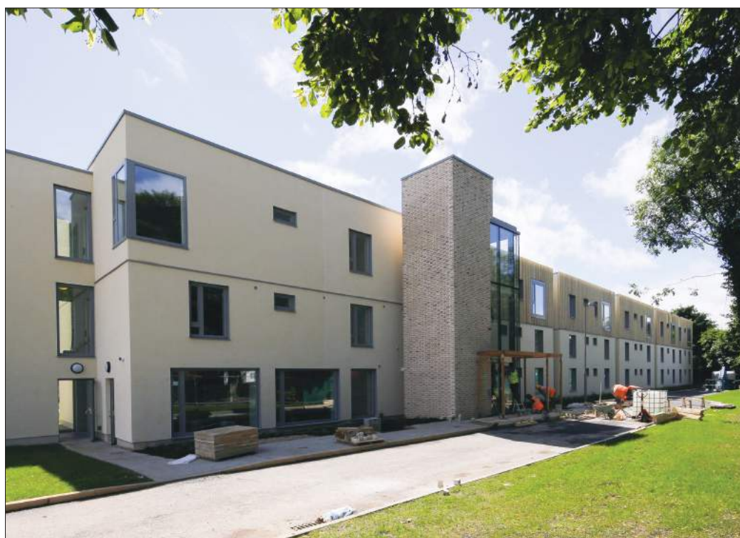
Works nearing completion at Rochestown House Phase 2
