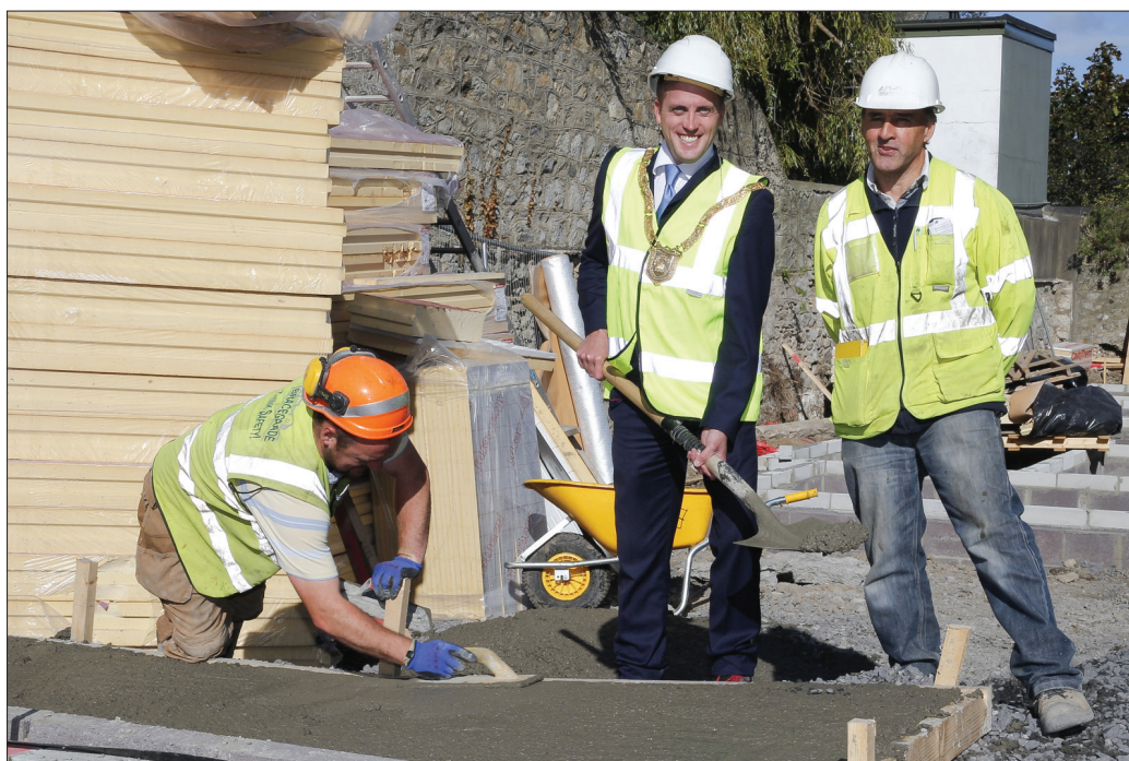
An Cathaoirleach, Cllr Cormac Devlin and contractors get works underway at St. Michael's Terrace
