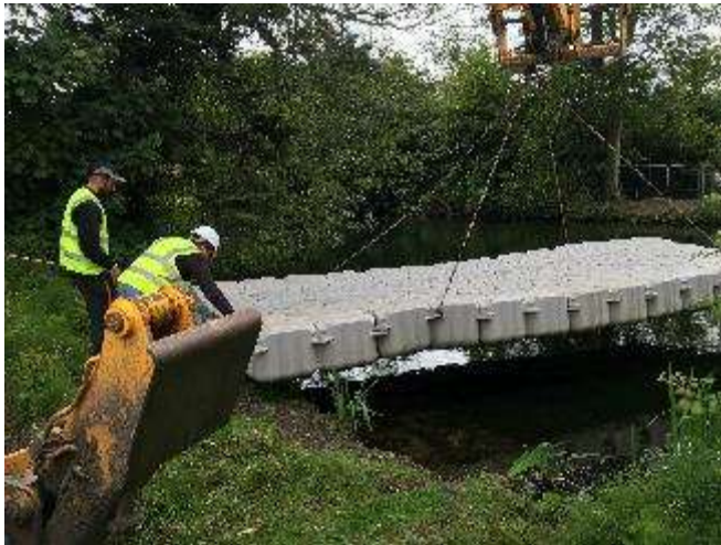
Plate 10: Monitoring of installation of Pontoon
