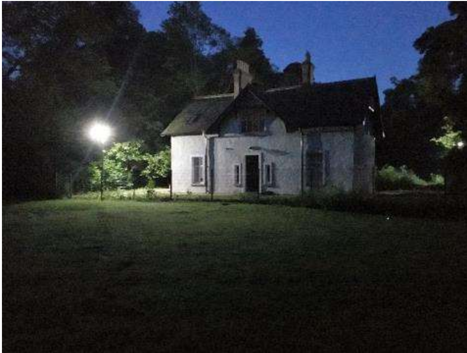
Plate 6: Security Lighting at Farm Yard buildings.
