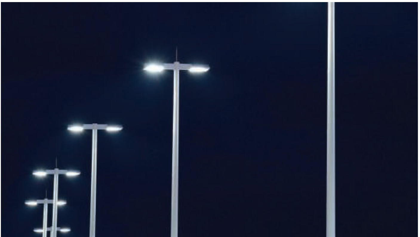
Above: public lighting
