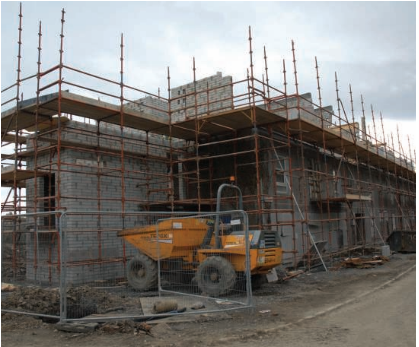
Below: Rochestown House Phase 2 Works
