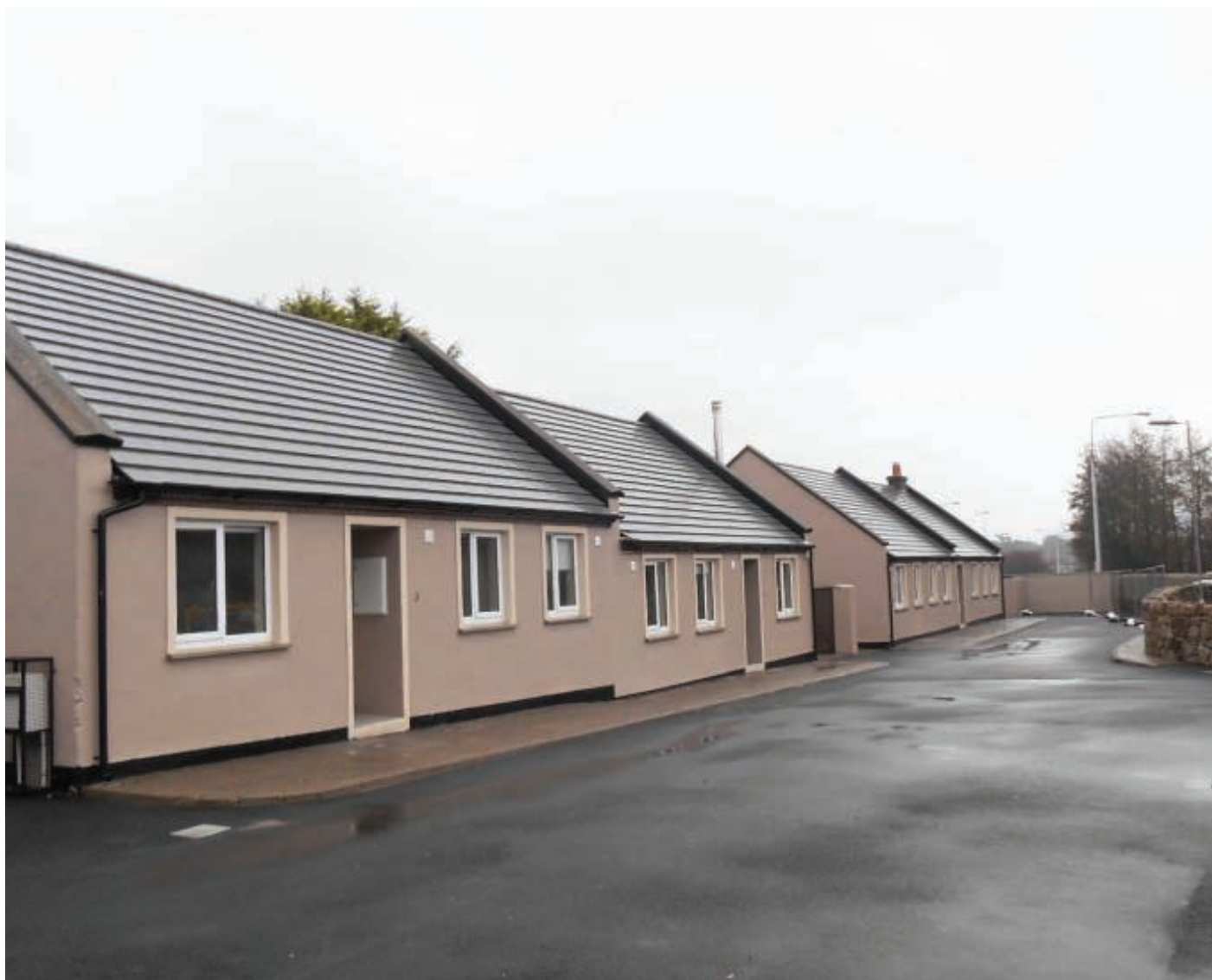
Below: Refurbished Traveller Accommodation Units at Glendruid Court
