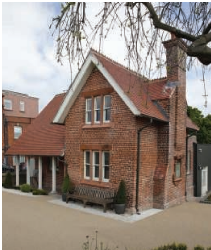
Below: Refurbished Gate Lodge
