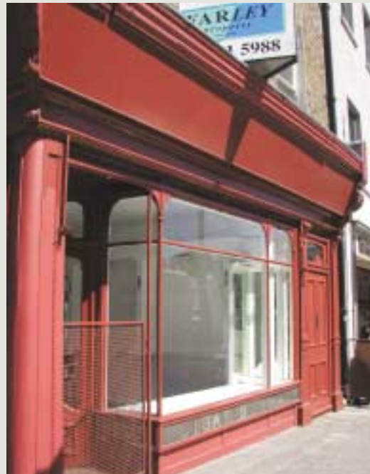
The essence of good repair work is to retain the maximum amount of viable fabric that contributes to the character of the shopfront, to carry out the work using proven methods of repair and to fit appropriately detailed new elements where necessary. This shopfront was carefully repaired with grant assistance from the local authority
