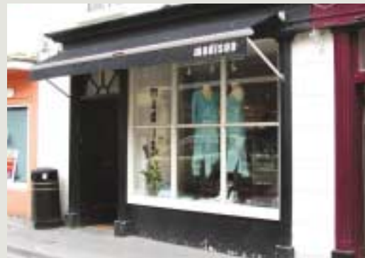
A new awning has been successfully fitted to this shopfront without the need for a visually obtrusive blind box
