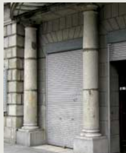
The entrance doors to this establishment have been fitted with roller shutters. Although the physical impact has been minimised, the closed shutters nonetheless have a large visual impact on the appearance of the structure and the streetscape. This impact can sometimes be overcome with the use of internal demountable grilles, a less visually obtrusive option of securing a historic shopfront, especially when painted a dark or neutral colour
