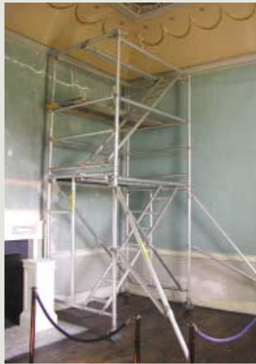
The erection and dismantling of scaffolding in rooms or spaces with important surface decoration or finishes requires especial care. Scaffolders experienced in such work may be required in these circumstances
