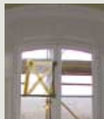
Glass is more vulnerable than most materials to damage during works, especially during the erection or dismantling of scaffolding. Historic glass should be protected at least to the exterior and, if necessary, also to the interior. Glazed windows should never be broken to facilitate scaffolding poles or ties, nor held open unless adequate protection is given to the glass and the sash is supported
