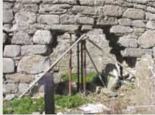
Structures may be in need of propping prior to, and during the course of, works which should be designed and installed to avoid causing damage to unstable fabric
