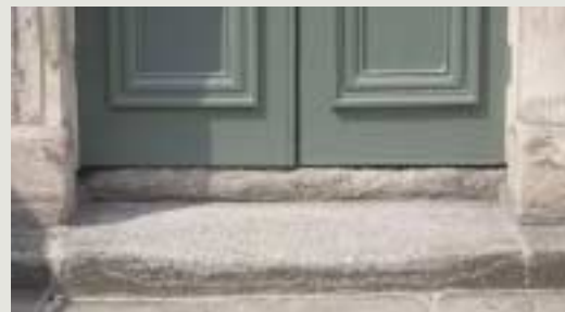
Traditional buildings almost always include one or more steps at the entrance, which may be important to the composition of the entrance and make a contribution to the character of the structure in the way they have worn through use over several generations. In the example shown here, the narrow double-leaf door would also cause difficulties for some disabled users but is essential to the character of the entrance
