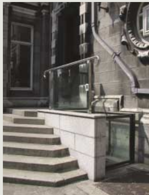
A well-designed platform lift of a sympathetic design using high quality materials, and provided in addition to, and not as a replacement for, steps may be acceptable. However, alternative solutions may have to be explored where a symmetrical or harmonious composition would be unbalanced or damaged by the addition of a ramp
