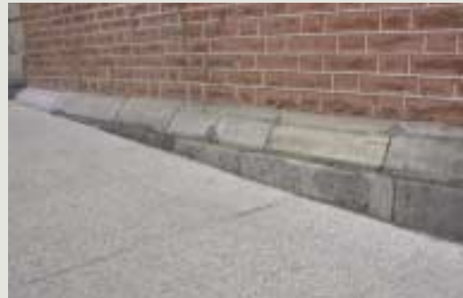
Access ramps against the façade of a building can conflict with or obscure important architectural features such as stone plinths. While a ramp may be physically separated from the masonry by a barrier to allow its removal without damage, the visual impact still needs to be resolved
