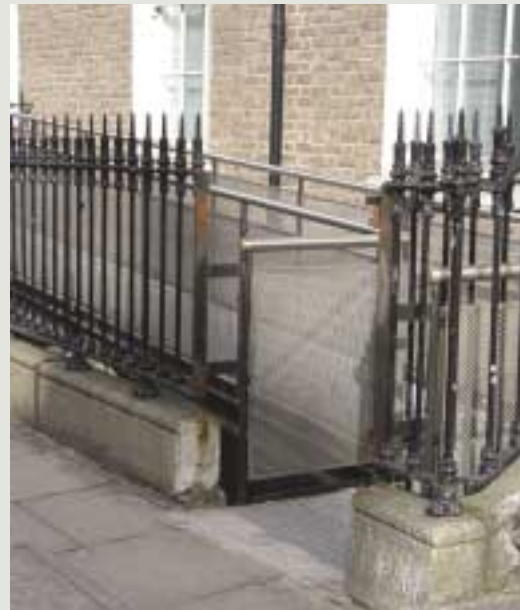
The traditional Georgian terraced house with a basement area to the front can present problems with regard to improving access. Alterations to provide a ramp can result in the loss or disruption of historic fabric such as stone plinths, iron gates and railings and can compromise the natural ventilation and lighting of basement rooms.
