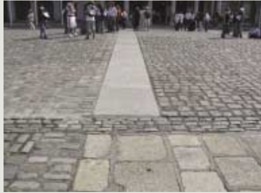
Traditional surfaces finishes can cause problems for those in wheelchairs or with walking difficulties but accessible routes can be provided through these areas using complementary materials
