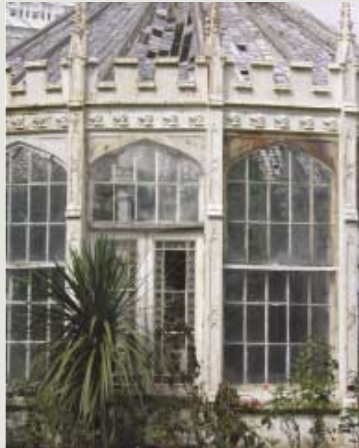
While it may sometimes be necessary to carefully dismantle an ironwork structure for repairs, some structures may consist of iron-clad sections on timber and masonry supports and may be more difficult to successfully dismantle and reassemble
