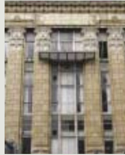
Terracotta, faience and glazed ceramic tiles are all used to good visual effect in cladding or decorating the walls of buildings
