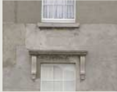
Localised re-rendering should be carefully specified to match the existing material. In this example, while the strength and texture may be adequate, the unmatched colouring of several patches is visually obtrusive
