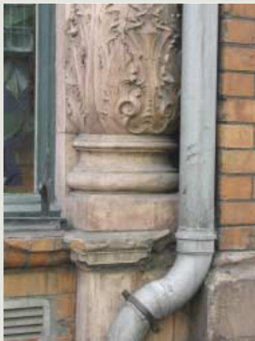
The ill-considered fixing of new items such as pipework to the principal elevations of structures can adversely affect their architectural quality and cause physical and irreversible damage, as has happened in this case where a fine architectural element has been cut through to facilitate the location of a new pipe
