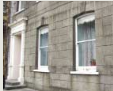
Render is a traditional coating which contributes both to the weathering performance and appearance of a structure. This house has been partially faced in Roman cement in imitation of rusticated ashlar and, while not the original finish, clearly contributes to its character
