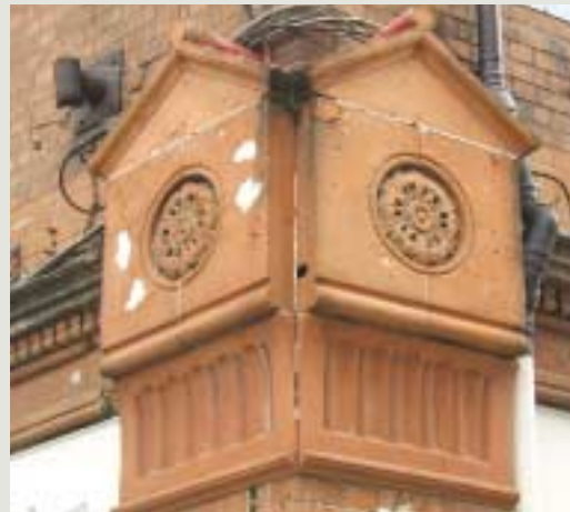
Materials such as terracotta and faience tend to be very durable. However, they can be damaged by aggressive cleaning methods. In this case, a later paint finish, together with the original fireskin of the terracotta, have been removed, exposing mortar repairs and old defects and leaving the ceramic vulnerable to future accelerated weathering
