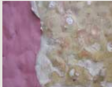
The way that limewashed render weathers contributes greatly to the patina of age: as it rubs away layers of different colours may be exposed. New coats of limewash can be applied as necessary without removing the existing layers
