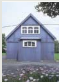
Metal sheeting consisting of flat or corrugated panels of iron, steel, lead, copper or zinc was used to clad many types of buildings, including places of worship such as this small church. Early metal sheeting is often of technical interest and should be identified and, where necessary, repaired, unless an inherent design fault requires its replacement to an improved specification
