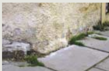
The injection of a damp-proof course may result in visually obtrusive pockmarks on the external walls of the building and is unlikely to be fully effective in rubble walling
