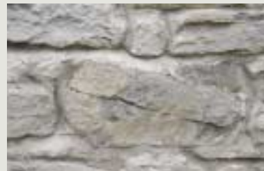
Even durable stones such as granite and limestone can be irreparably damaged by inappropriate works. The cement mortar used in repointing this wall is stronger than the stonework. As a result, structural movement in the wall could not be absorbed by the mortar and instead the stone has fractured. The impermeability of the mortar may cause future additional damage, as any water entering the wall through this fracture will be unable to escape
