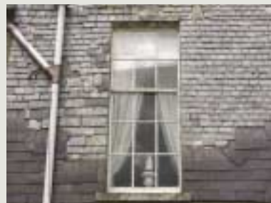
Slate-hanging should be carefully repaired where necessary using slates of a matching size and colour, with additions such as downpipes and vents carefully sited and fixed in order not to cause damage
