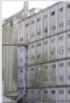
Early mass- and reinforced-concrete structures, as well as early blockwork and cast or reconstituted 'stone' structures may be of technical interest. This silo of 1905 is constructed of reinforced concrete using the pioneering Hennebique technique and is one of the few such structures surviving in Ireland
