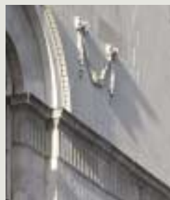
Coade stone, a proprietary fired clay, was used for fine decorative detailing. It generally makes a significant contribution to the character of the structure it adorns
