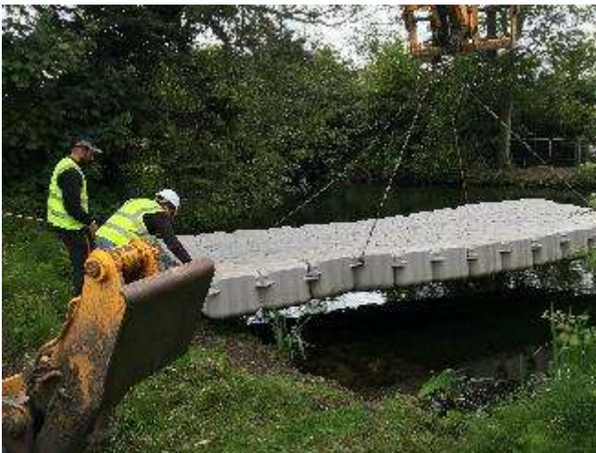
Plate 8: Monitoring of installation of Pontoon
