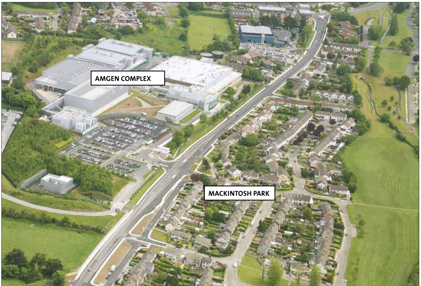
Aerial view of the new Pottery Road
