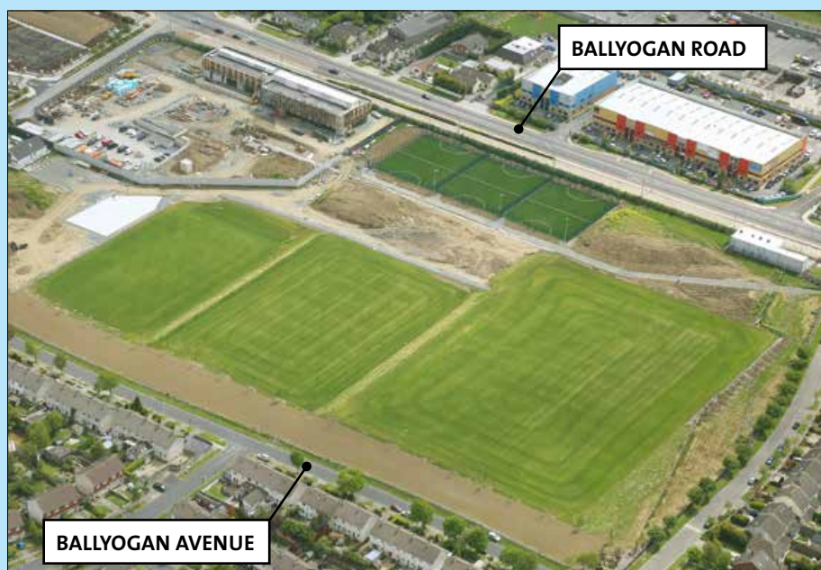
Aerial view of the Samuel Beckett Civic Campus
