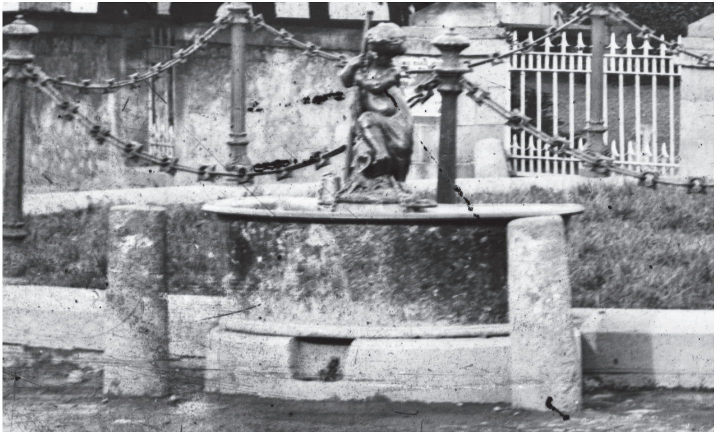
Detail of the c1890s photograph from the Lawrence Collection showing the bollards and cherub at the trough
