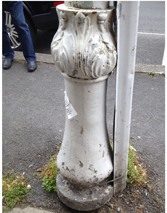
The existing bases to the former tram masts which have been reused for light poles are to be carefully removed and stored for later use
