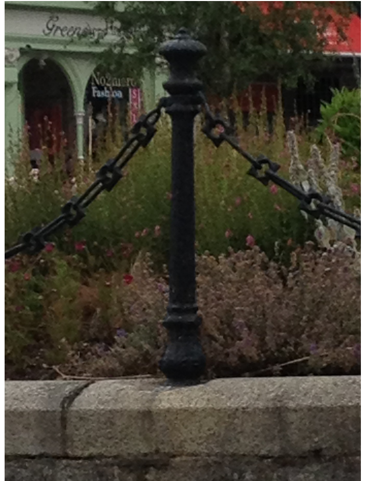
View of cast iron post on granite base with cast and wrought iron chain.
