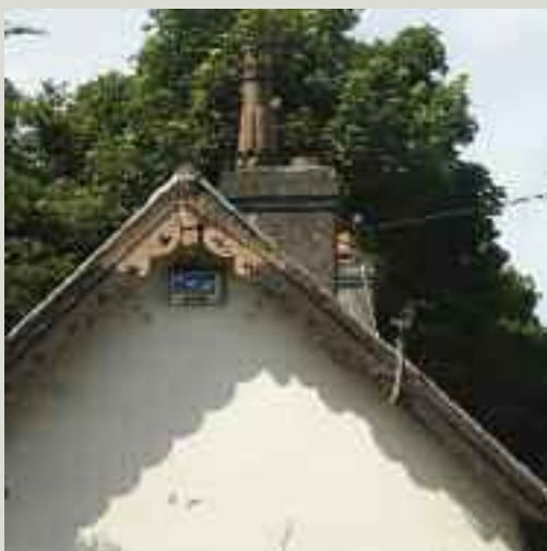
The poor condition of overhanging verges can lead to deterioration of the ends of the purlins as well as the loss of sections of decorative timber bargeboards
