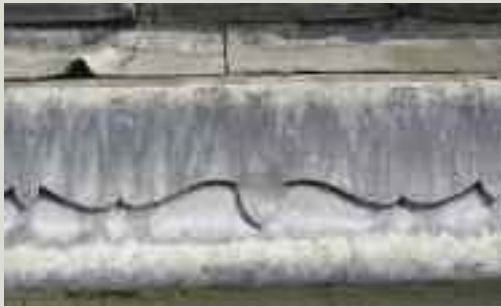
In high-quality work, the visible edges of lead flashings were cut to decorative shapes
