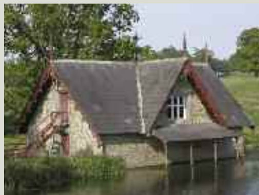
The overhanging gable detail comprised an extended roof to protect the masonry gable and was finished with bargeboards which could be decorated and painted
