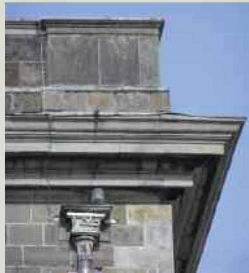
A rare example of a surviving lead hopper head with an embossed date of 1725
