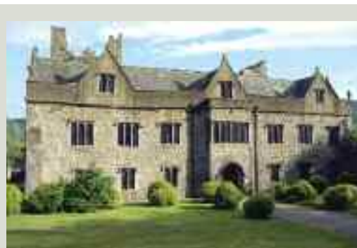
Tower houses were heavily fortified, with their roofs concealed behind battlements. In contrast, the architecture of the sixteenth and seventeenth centuries brought the roofscape increasingly into full view. At Ormond Castle, County Tipperary, the remains of the earlier tower house can be seen rising behind the Elizabethan mansion with its then highly fashionable dormer gables
