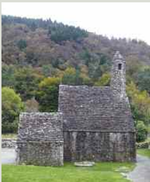
Saint Kevin's Church, Glendalough, County Wicklow. The steeply pitched roof of local stone was built up by corbelling and is supported on walls almost 4 feet (1.2m) thick
