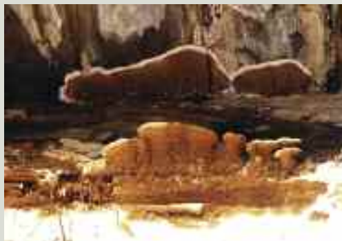
The fruiting bodies of the serpula lacrymans fungus can be identified by their rust or orange colour, usually with a white edging
