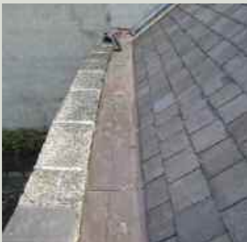
Parapet gutter re-lined in copper. The very shallow falls to this gutter precluded the use of lead
