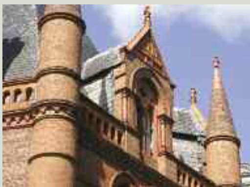
Victorian roofs are often architecturally complex, using a variety of roof shapes, roofing materials and embellishments
