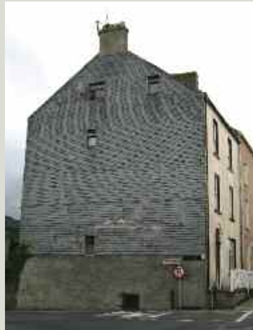
The best surviving examples of native Irish slate are most often found in vertical slate hanging, as it requires less frequent replacement than roofing slate. It is thought that this example of a slated gable is covered in Ahenny slate from the nearby Ormond quarries in the Carrick-on-Suir area
