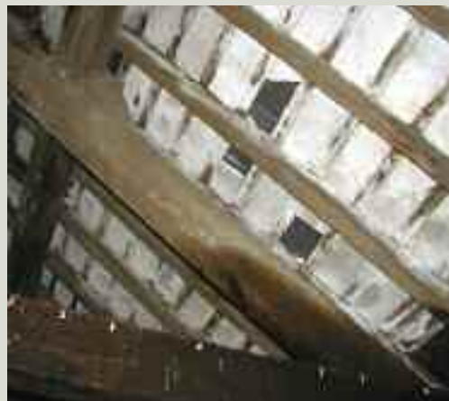
Substantially intact parging to the underside of slates is visible from within the attic space and provides a secondary line of defence against rain and wind entering the interior of the building
