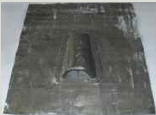
An especially formed lead vent with fly mesh, for use on a church roof. As they are quite distinctive and visible, the use of these vents on a roof where none existed previously should be discussed with the architectural conservation officer in the local authority
