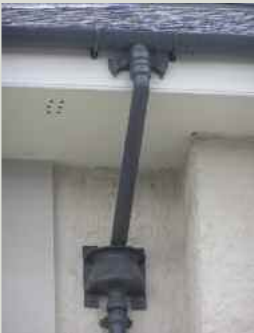
Cast-iron rainwater systems often copied the design of leadwork, but the stronger nature of cast iron enabled the use of shallow collars and two-point fixings rather than the deep collars needed to support lead rainwater goods
