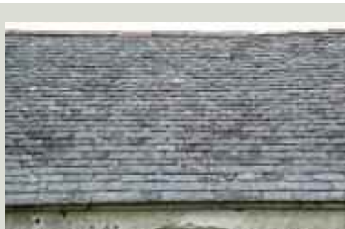
An example of a gauged roof of Ahenny slate, where the sizes of the slate courses gradually get smaller, or diminish, towards the ridge of the roof
