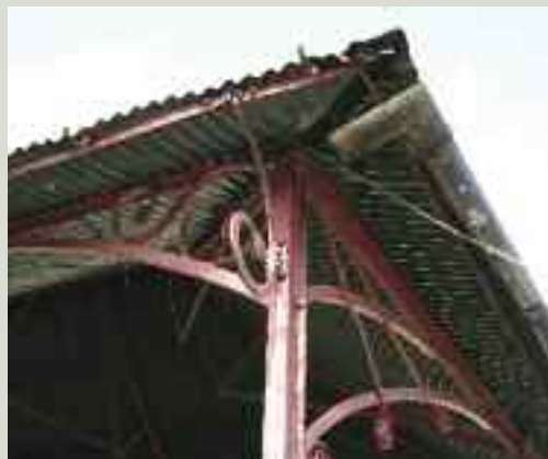
This corrugated iron is suffering from pitting, visible as small pinpricks of light where the metal has corroded through. There is also crevice corrosion occurring at the junction of the sheet with the hip roll. In addition, work is urgently needed to repair the rainwater goods
