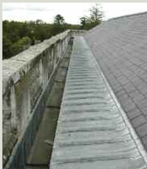
Welts to lead flashing to the vertical face of the parapet wall. Note the steps in the lead gutter and the rolls in the lead apron on the lower portion of the roof slope
