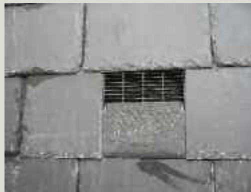
Example of an in-line slate vent. The vent will not protrude above the roof plane. However, such vents may be unacceptably conspicuous if used on the outward-facing slopes of a roof
