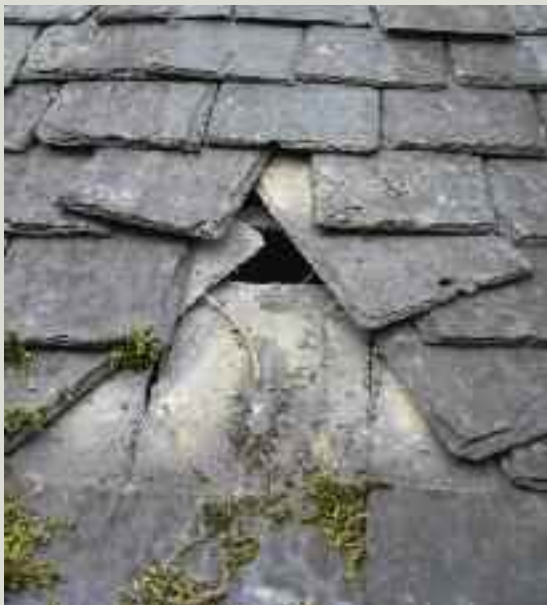
Earlier slate roofs using top-hung, single-nailed slates can easily be repaired by swinging individual slates aside allowing access to replace or re-peg the slates beneath
