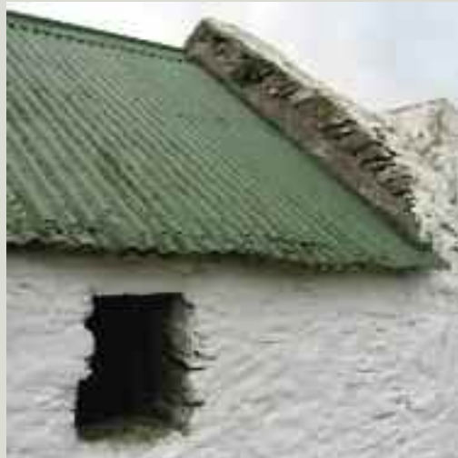
The eaves edge of corrugated-iron sheeting is particularly vulnerable to corrosion. Here, additional layers have been inserted under the eaves
