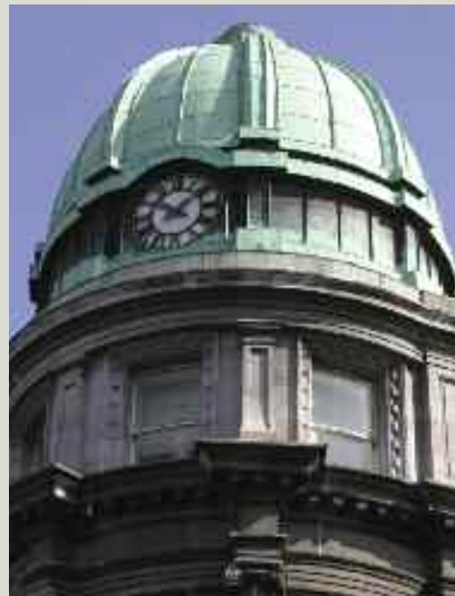
Copper was used to clad eye-catching architectural features on buildings, embellishing elements such as cupolas, domes and steeples
