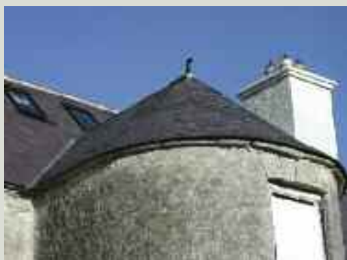
The repair of curved slate roofs is highly specialised work and requires a roofing contractor who has experience and skill in gauged work
