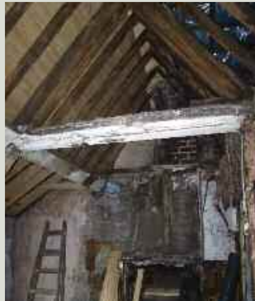
An early-seventeenth century roof showing the original principal roof structure and rafters with replacement sarking boards above (Image courtesy of Tom McGimsey, Mesh Architects)
