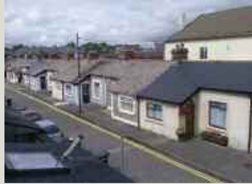
The mix of roofing materials on this terrace of houses visually fragments its appearance. The use of 'artificial slate', or fibre-cement tile is visible in the foreground, and also further down the street, striking discordant notes among the original slate-covered roofs
