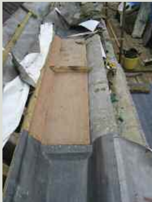
The design of this parapet gutter has been revised to achieve correct lead sheet lengths, falls and step heights in order to ensure that the newly-laid gutter will achieve a good lifespan. Note that the lead sheets have been fixed at the top end only (to allow for expansion and contraction), using copper nails in a staggered pattern
