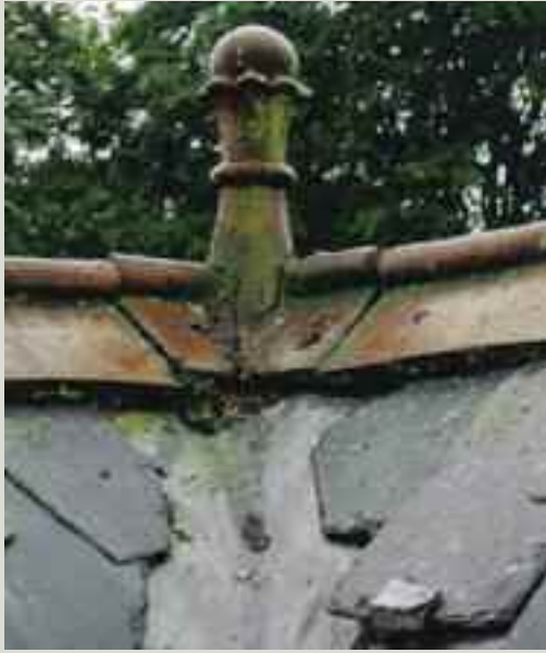
This terracotta ball finial was cracked; as part of a roof repair project it was removed, carefully cleaned and repaired before re-installment
