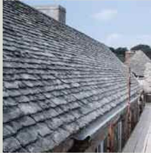
A new flush eaves gutter formed in lead along the top of the wall
