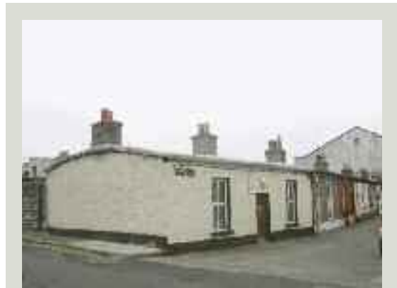
The 'Portlaw' roof was also used further afield for housing schemes, such as here in Harold's Cross, Dublin; also in Clara, County Offaly; Blarney, County Cork; and Carrick-on-Suir, County Tipperary. At one point, these trusses were exported to Germany
