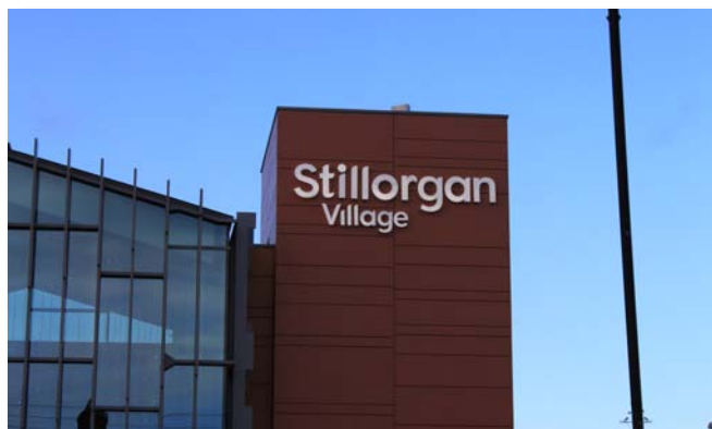
Photo 10: New sign at Stillorgan Shopping Centre
