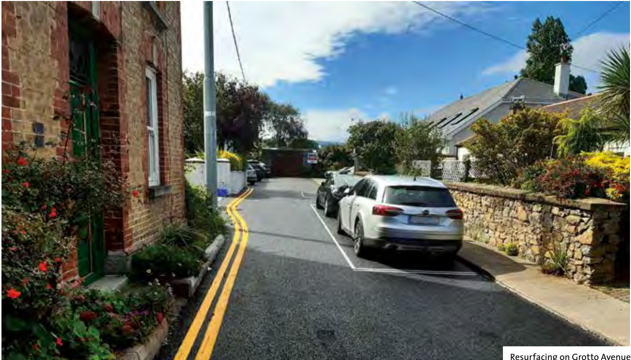
Resurfacing on Grotto Avenue
