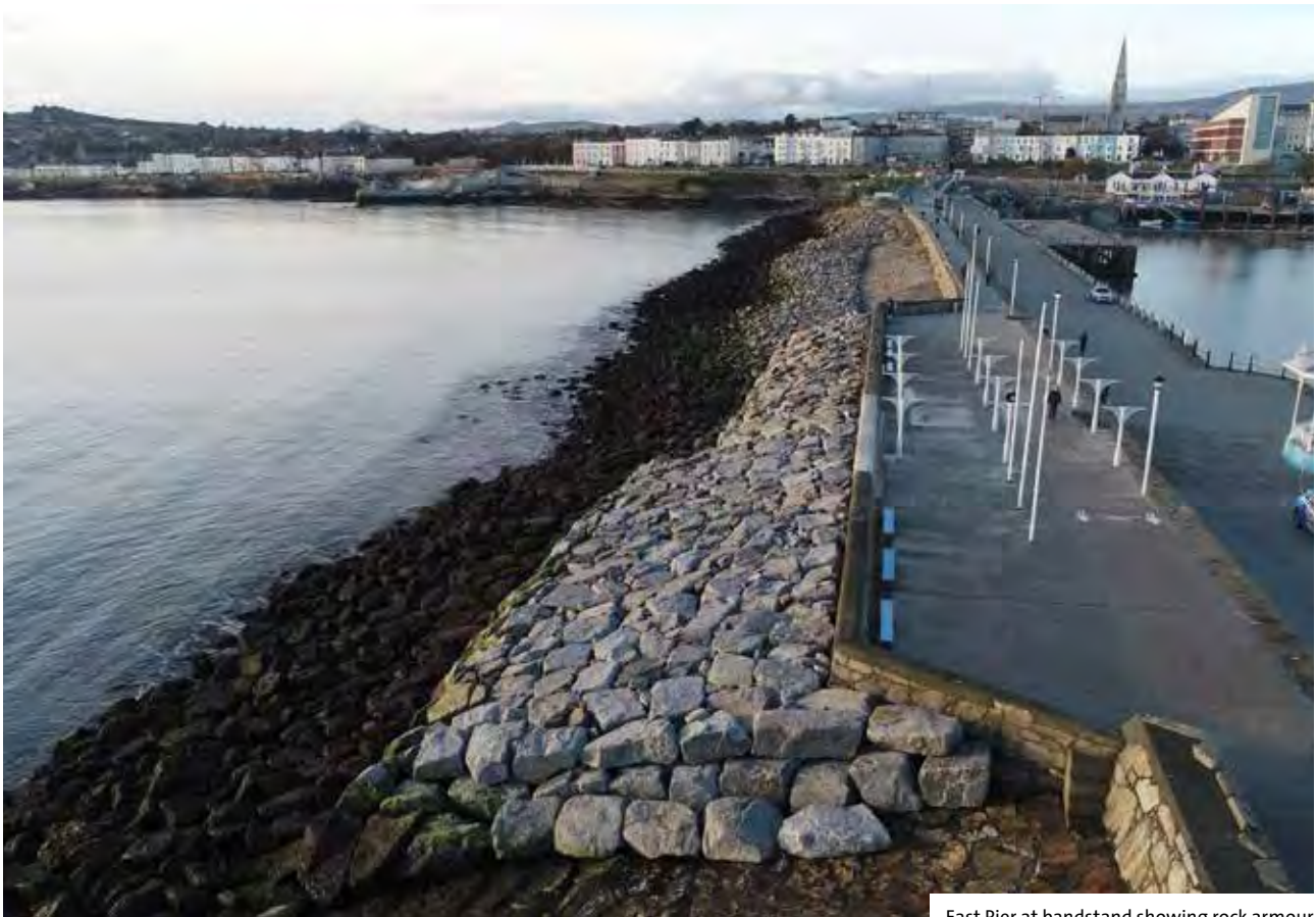
East Pier at bandstand showing rock armour
