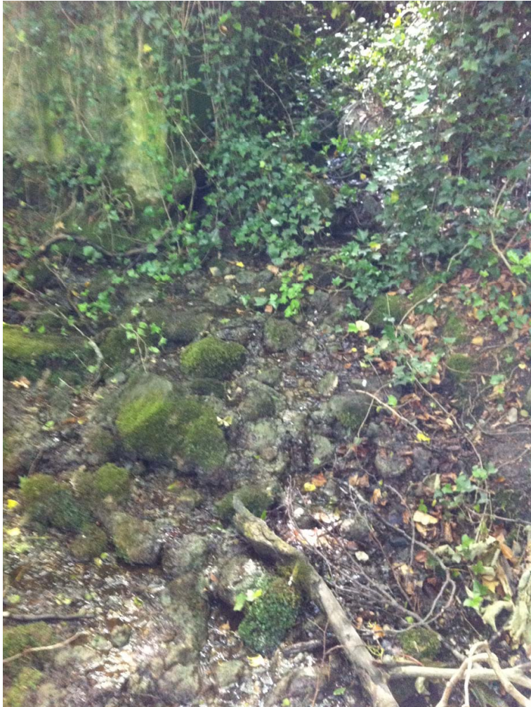
Photograph 5 –Tuffa formation along drainage stream from spring emergence at location 11. Concrete water holding tank visible at top left corner of image.
