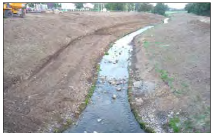
Construction Stage of Flood Alleviation at Deansgrange Stream
