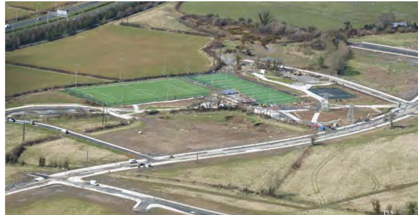
Western aerial view of infrastructure works at Cherrywood
