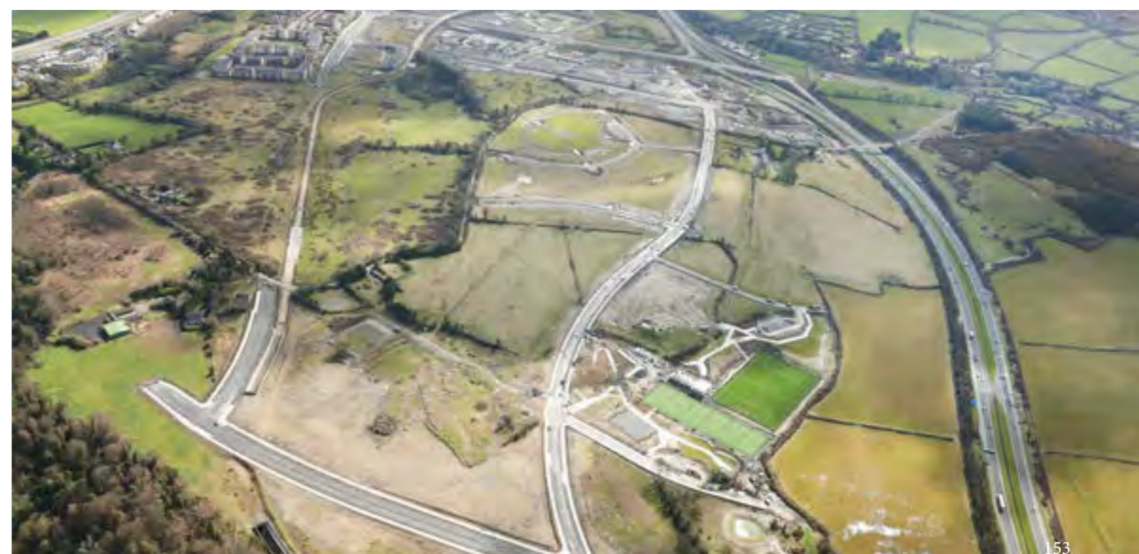
Southern aerial view of infrastructure works at Cherrywood
