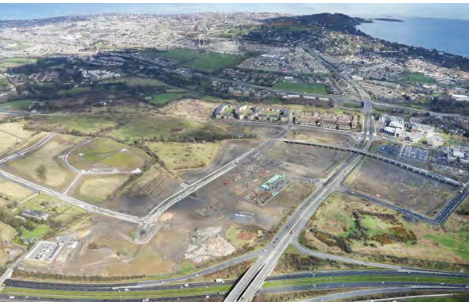
Northern aerial view of infrastructure works at Cherrywood
