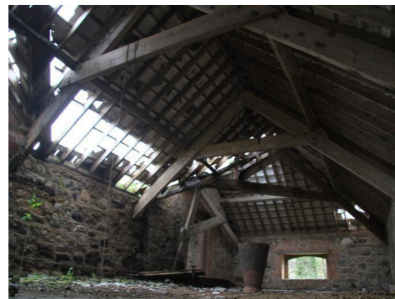
Above: Hay loft with A-truss timber roof
