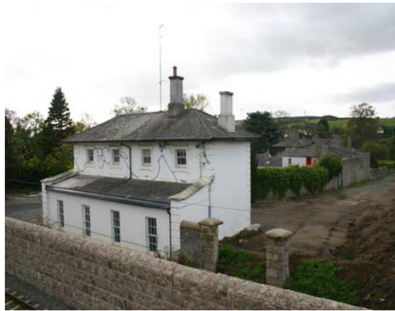
Above: Northern view of building
