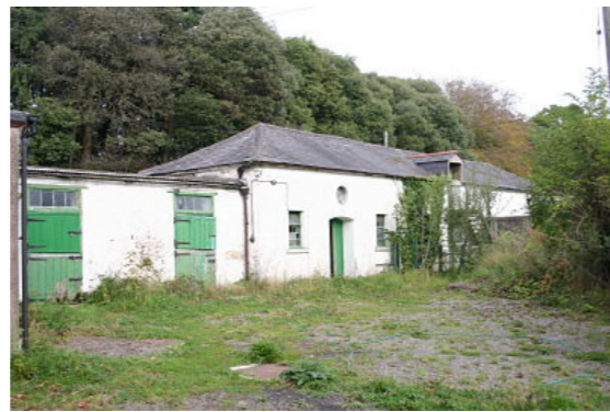
Above: Stables on western side of yard
