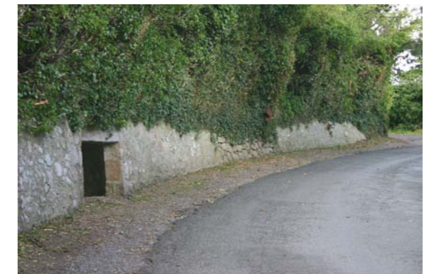
Above: Possible well, Lehaunstown Lane
