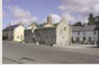
In this instance, a ruined markethouse marks the centre of a planned village. Despite its ruined state it forms a local landmark which, if lost, would remove the focus of the historic townscape
