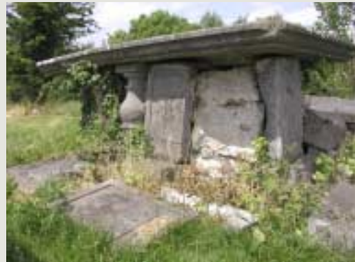
While there is generally a respect in communities for burial grounds, the wish to maintain them should not lead to over-enthusiastic or misguided 'tidying-up' works or the uninformed reconstruction of damaged memorials. Where repairs are planned to damaged memorials, all fragments should be identified and reset using an appropriate mortar, and any poorly executed previous repairs rectified, if this can be achieved without further damage. Specialist advice will usually be required
