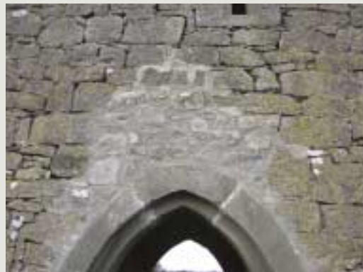
Care should be taken to match repairs to the existing in terms of materials and workmanship. This mediaeval doorway was rebuilt using an inappropriate cement mortar. The stones above the point of the arch have been set in a random pattern and finished with wide joints quite unlike the surrounding stonework
