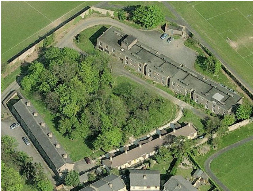
Existing buildings on site
