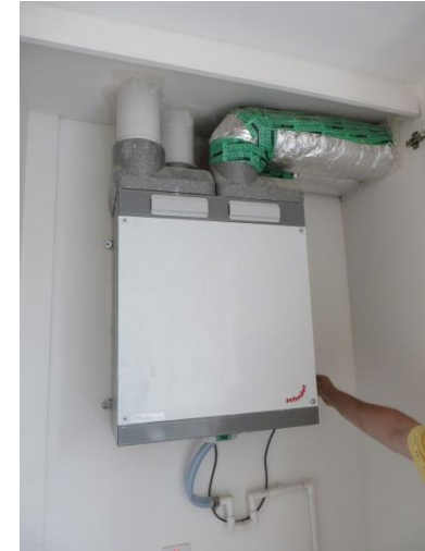
Heat Recovery Ventilation
