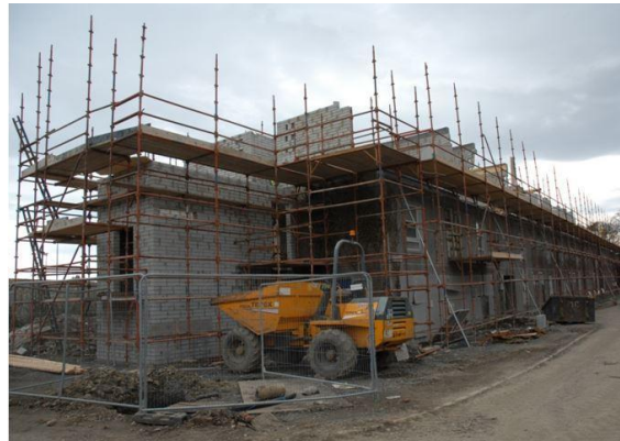
2 nd floor extension
