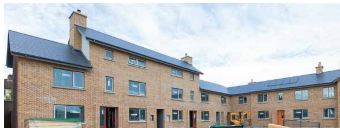
New homes being constructed at Fitzgerald Park.
