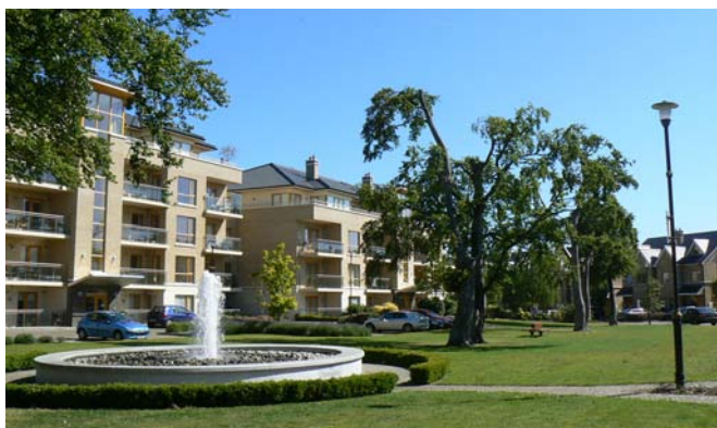
Photo : 2 Development at Trimbleston, Goatstown
