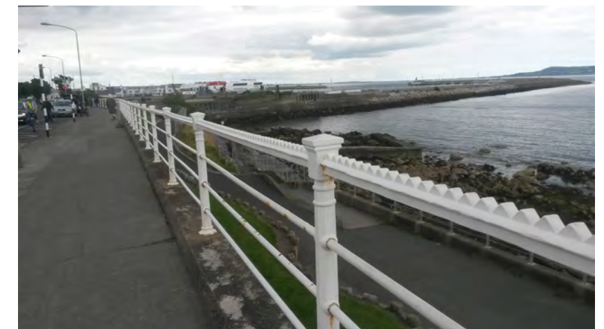
Photo 25: Railings along Queen's Road, Dún Laoghaire.
