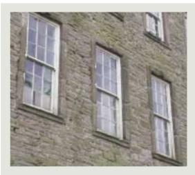
These windows are pictured prior to a recent repair. While it was initially thought rails, sills or stiles would need replacement or splicing-in, on examination very little timber repair was required. The crown and cylinder sheet glass was retained in the repair and redecoration works. It is important to inspect all historic elements on an individual basis prior to specifying works, in order to ensure that only necessary repairs and replacement of parts are carried out
