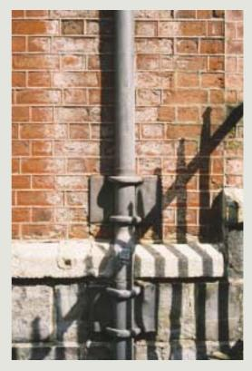
It is good management practice to regularly inspect a structure to ensure that rainwater continues to drain effectively. In this case a blockage in a new lead downpipe resulted in overspill onto the wall behind, which was not remedied in time to prevent efflorescence occurring on the face of the saturated brickwork
