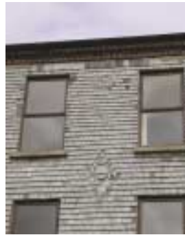
Conscious artistic input can bring special interest to otherwise ordinary structural elements such as slate-hanging, brickwork, chimneystacks or shopfronts within an area
