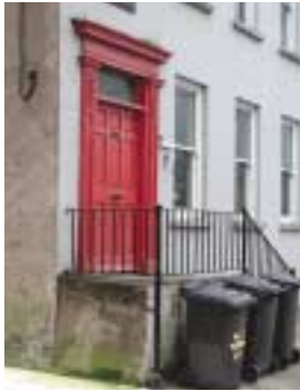
Consideration should be given to the storage of waste disposal bins as these can have a large visual impact on an area
