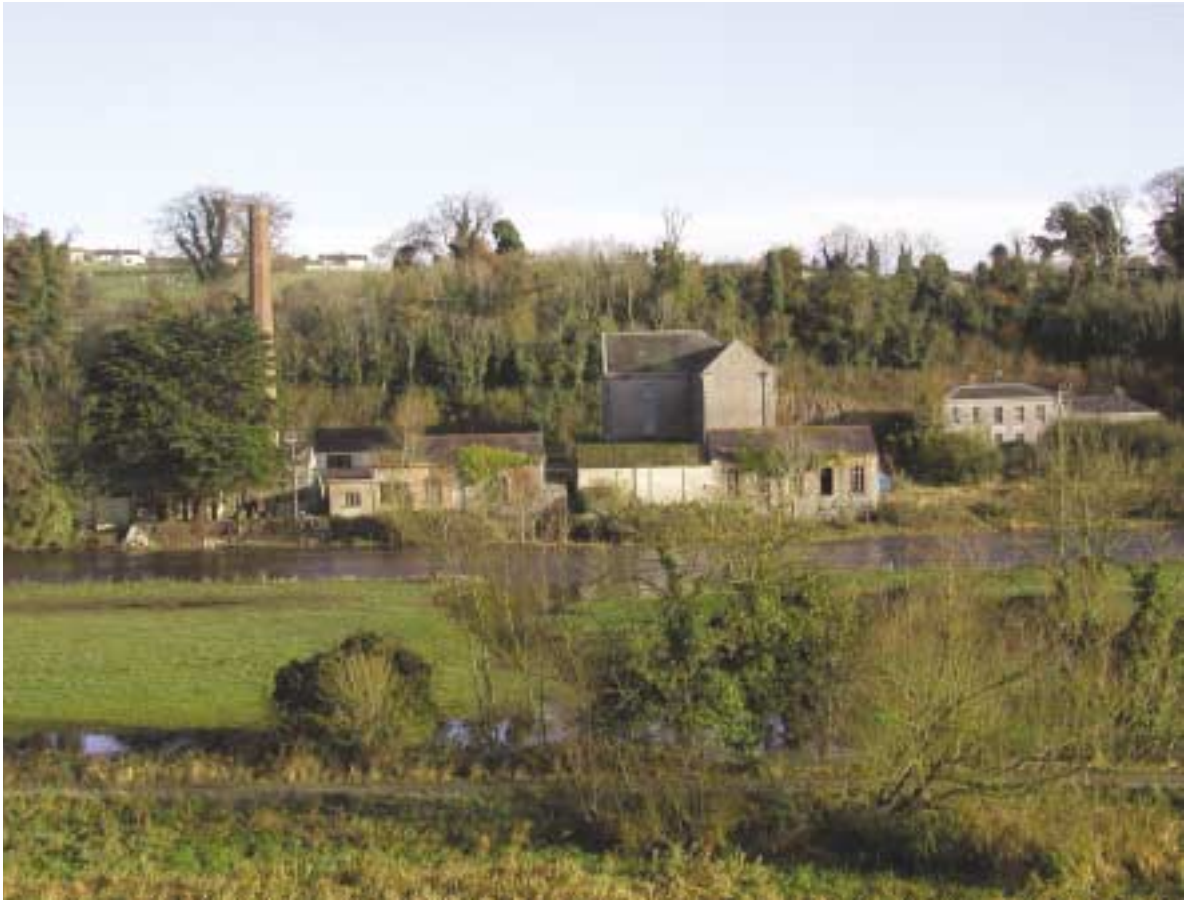
These mill buildings at Slane Bridge are of outstanding importance as an example of an early purpose-built industrial complex dating from the start of the Industrial Revolution
