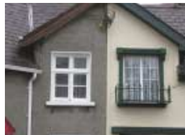
Inappropriate small-scale alterations may gradually make a significant impact on an area and erode its character
