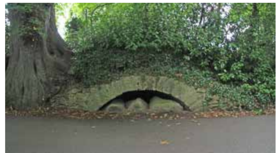
In filled under passage walkway, Marlay Park
