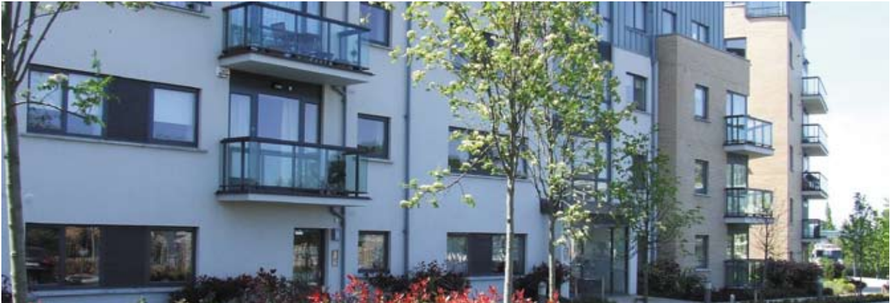
Wyckham Point, Ballinteer - one of the developments in which the Council is offering dwellings under the Affordable Housing Scheme
