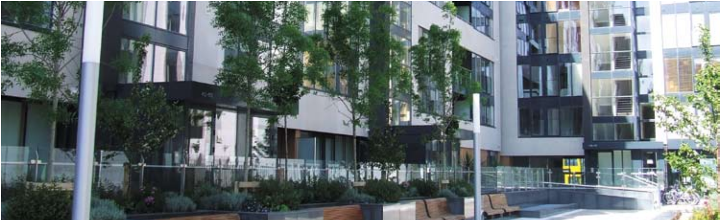
Harbour Square, Dun Laoghaire - a development where dwellings are available under the Affordable Housing Scheme
