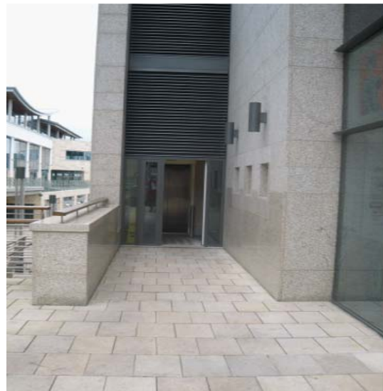
Photo 4.2 Access for All Elevators at Dundrum Shopping Centre
