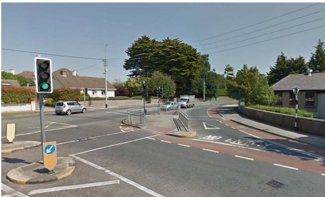
**Figure 7.14:** Limited footpath space, excessive road engineering and conflict between cyclists and vehicles.
