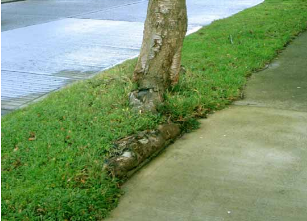
Footpaths are regularly replaced as a result of damage by Cherry tree roots
