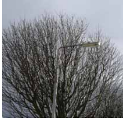
Tree interfering with public lighting
