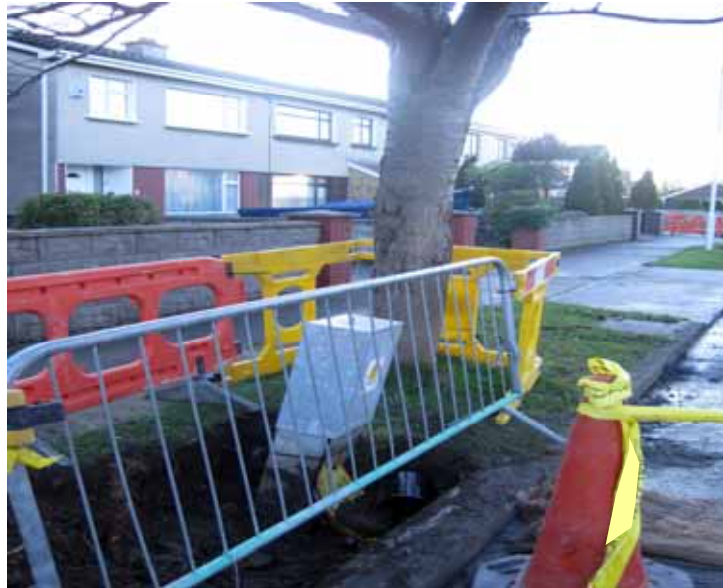
Utilities being installed close to a street tree
