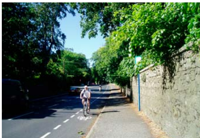
Photo 6: Cycle Lane on Old Dublin Road
