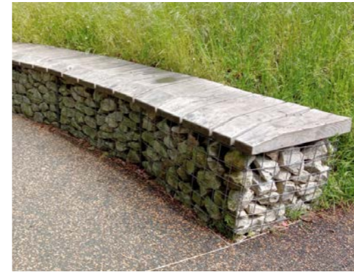
Gabion bench with timber top
