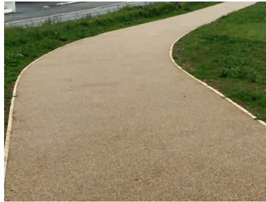
Provision for light buff, red and green pigmented bound gravel in cycleways.
