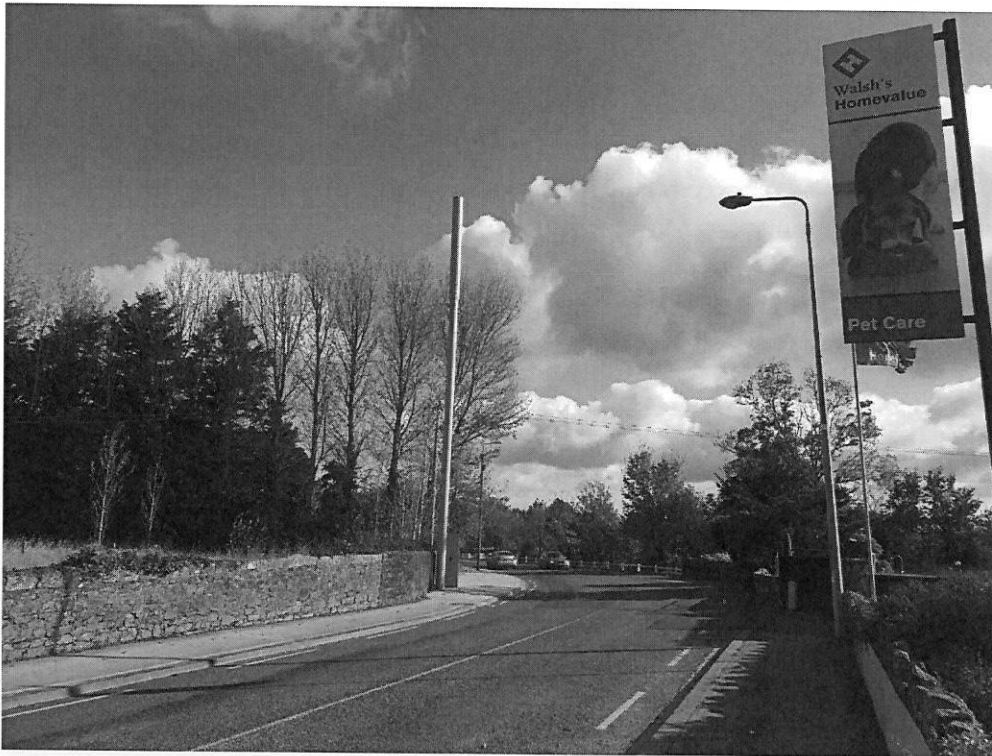
Fig 1. Existing 15m Smart Streetpole Solution as erected in Bagenalstown, Co Carlow
