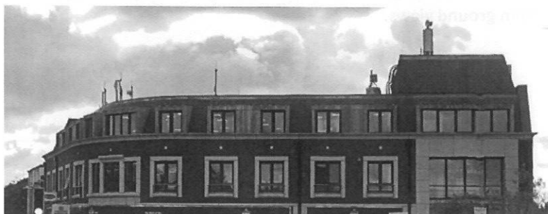
Image 5 Existing eir Mobile rooftop site (co-located) in Stillorgan ComReg Site ID: 1312
