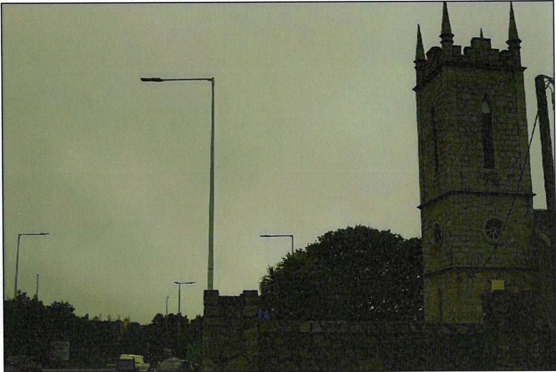
Image 3 Existing view S from entrance to St Matthias's Church (VP2, Photomontage Report, Entrust Planning & Environmental)
