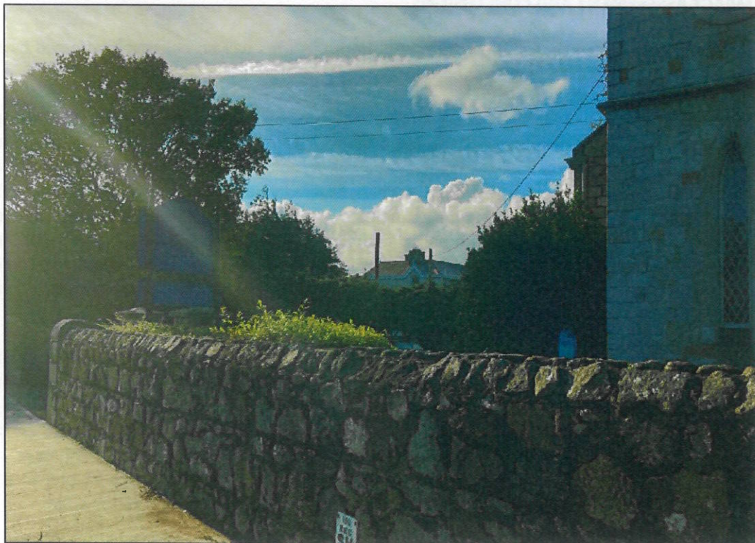
Plate 4 View of rooftop of Rectory (Woodfield) from roadside, at church boundary wall, facing SW
