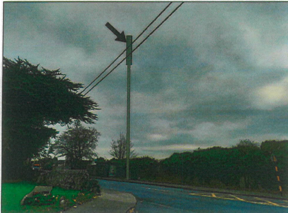
VRP1 - WITH SOLUTION IN PLACE
