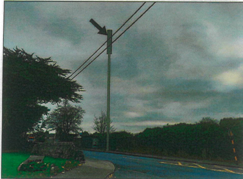
VRP1 - WITH SOLUTION IN PLACE
