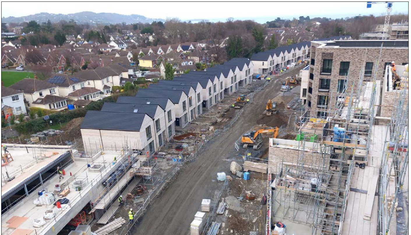
Shanganagh – construction progressing of 597 new homes in Shanganagh
