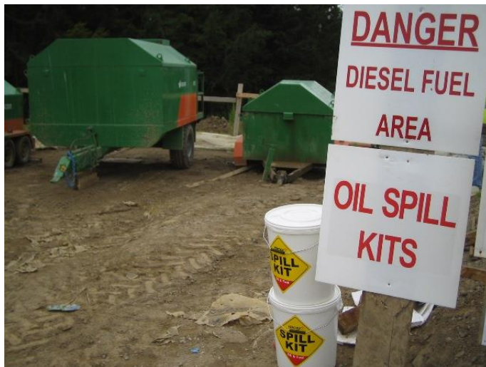
Photos 3 & 4: Spill kits located next to watercourses
