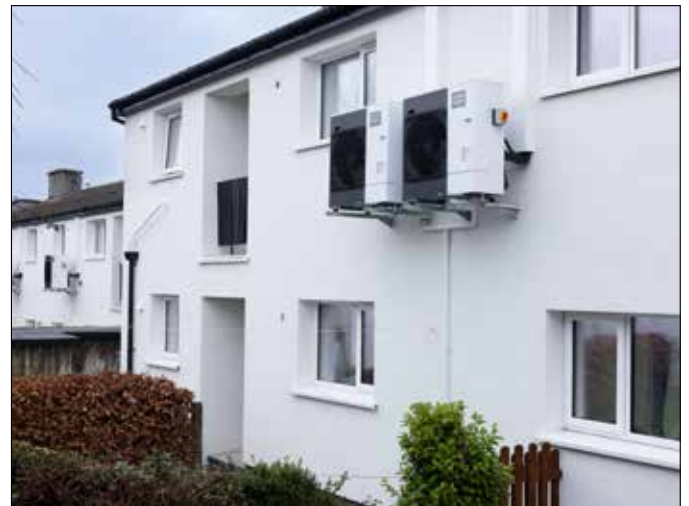
Glasson Court Retrofit – xxxx homes at Glasson Court retrofitted under the Energy Efficiency/Retrofit Programme
