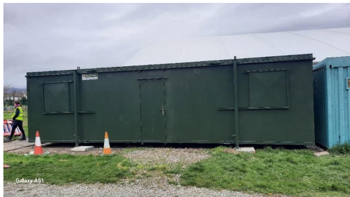
New unit dropped into place
