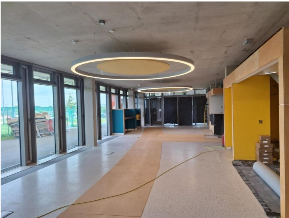
Above: Ground floor and entrance to new Ballyogan Library
