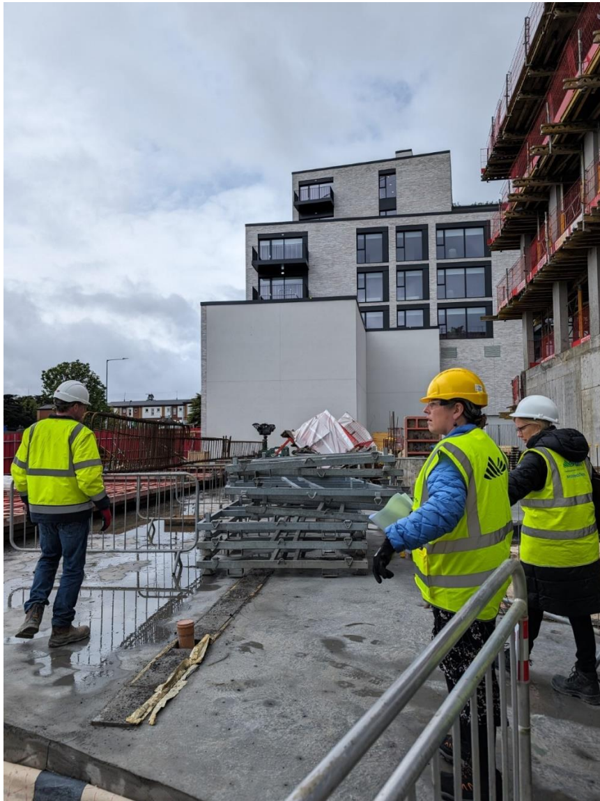
Above: Stillorgan Library redevelopment
