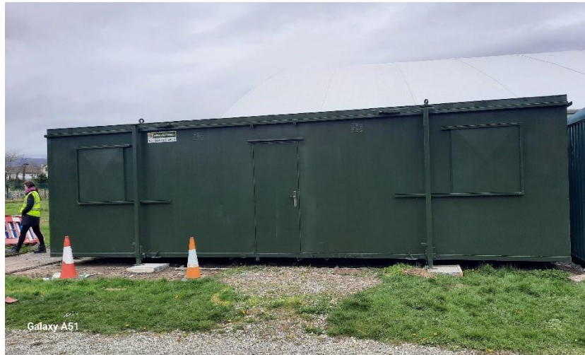
New unit dropped into place
