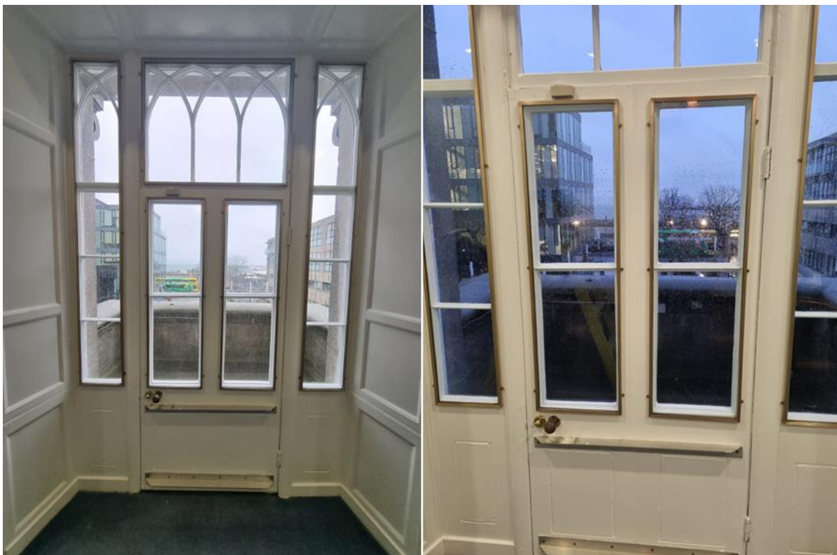
Figure 27 Laminate glass glazing panels on balcony doors
