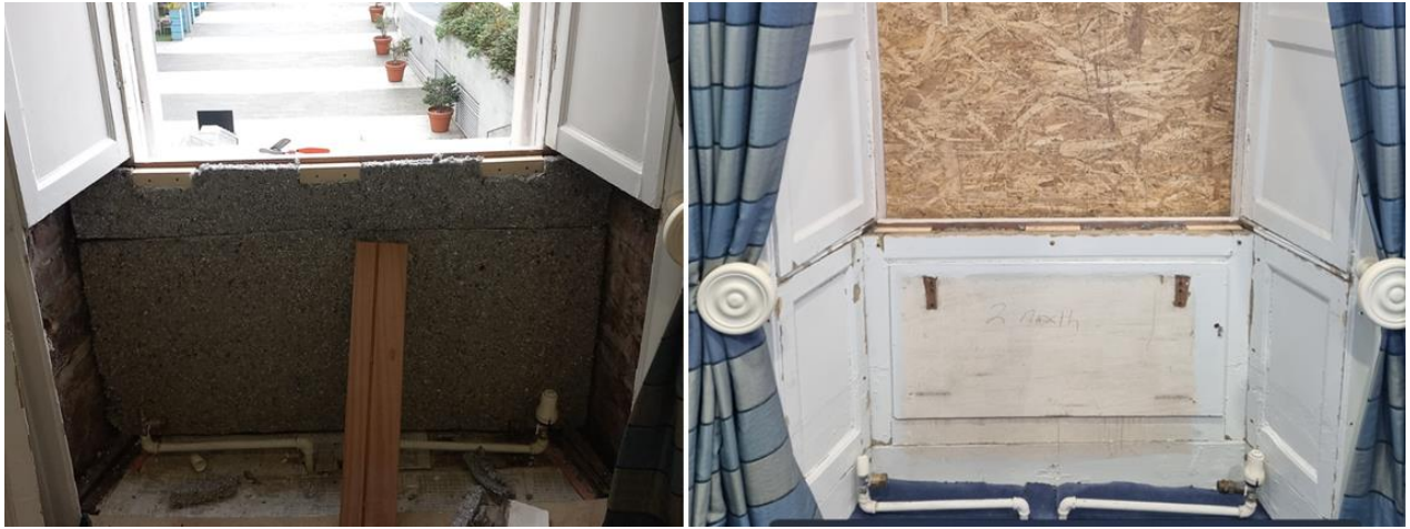
Figure 13 Boardroom window 2 north insulated with 70mm Pavacell & panel reinstalled
