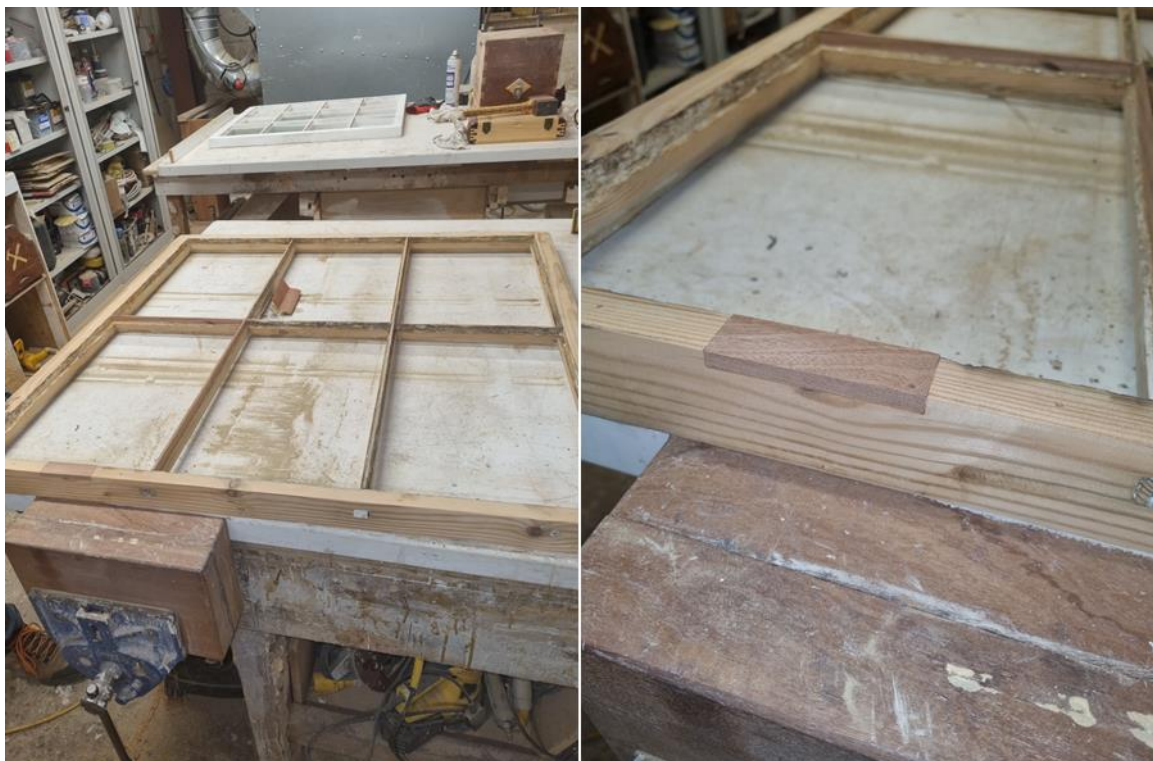
Figure 4 Frame & glazing bars repaired with Mahogany
