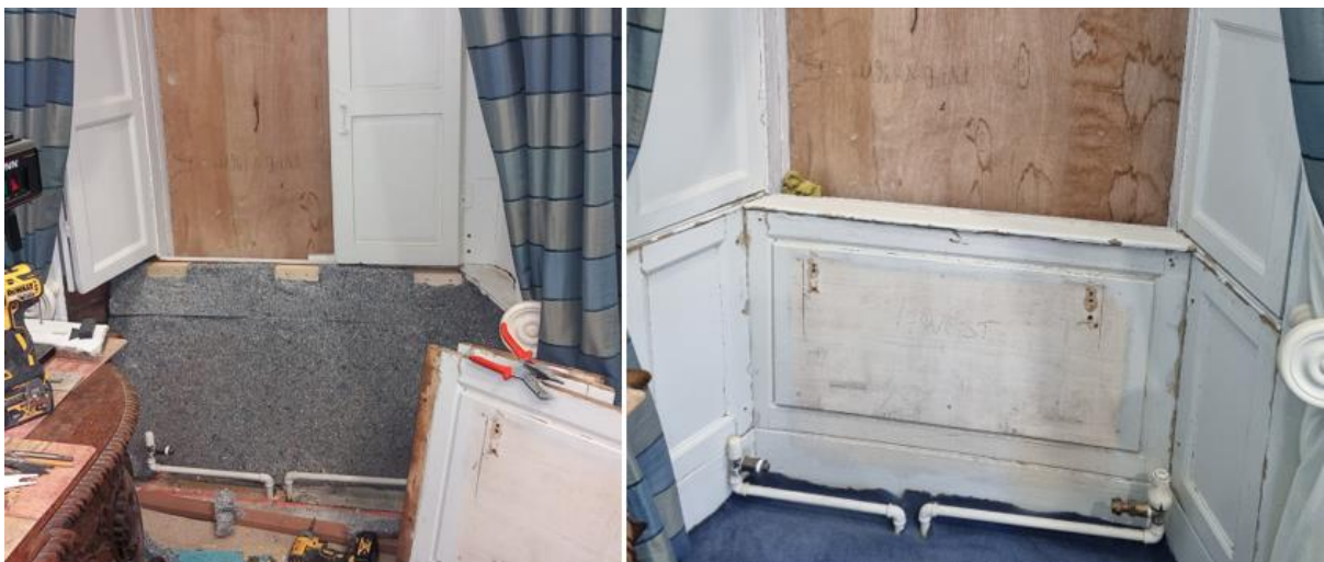
Figure 12 Boardroom window 1 west insulated with 50mm Pavacell & panel reinstalled
