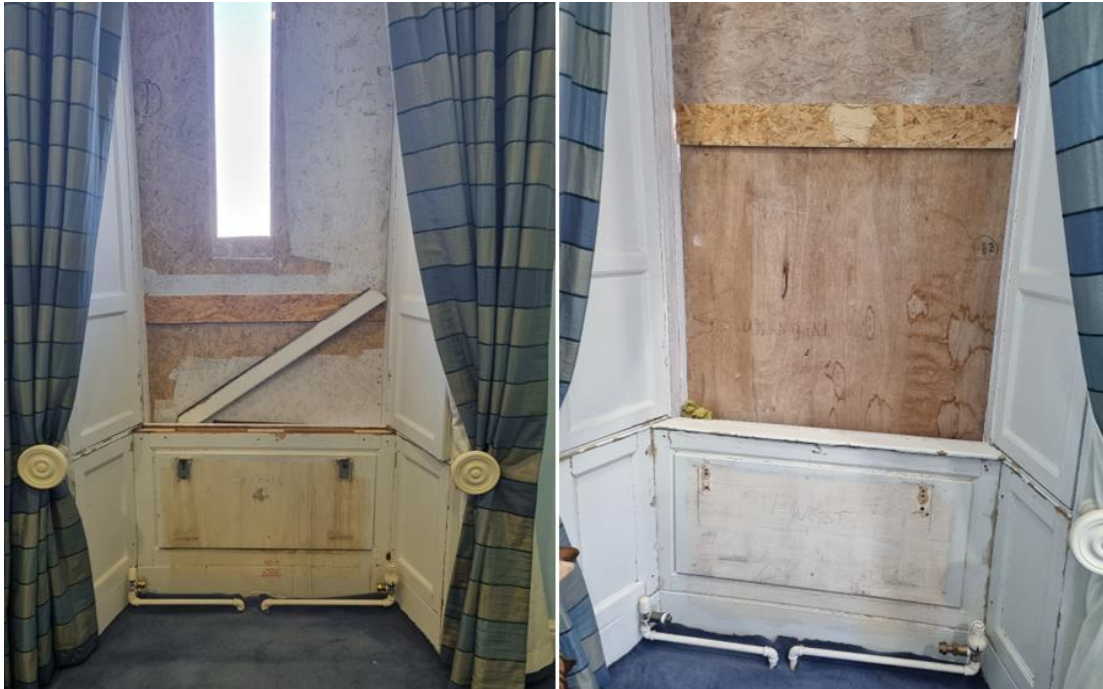
Figure 16 Window openings secured with ply
