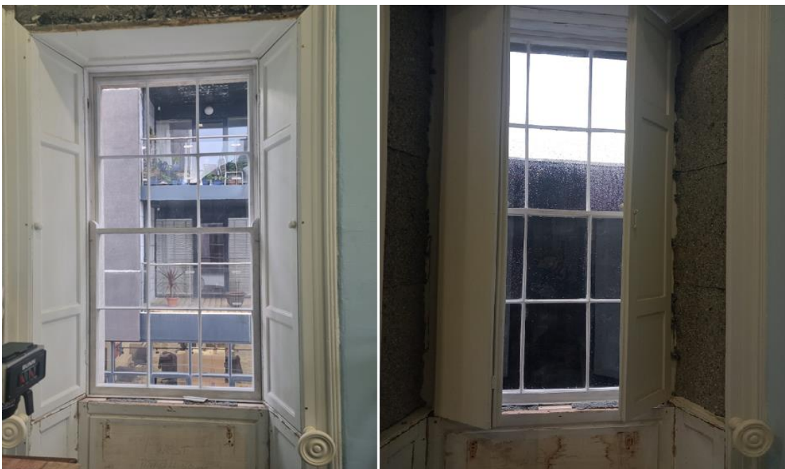
Figure 17 Original refurbished windows reinstalled in the boardroom
