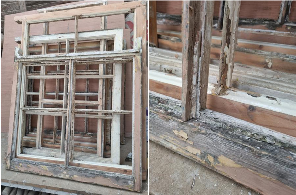
Figure 3 Frames cleared of putty and original glass
