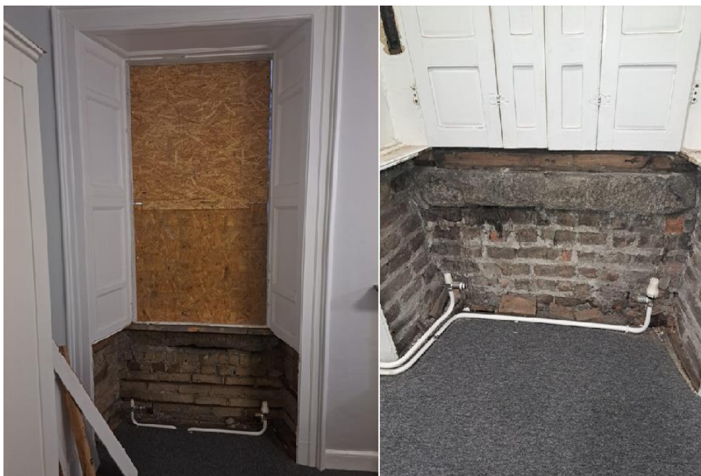
Figure 19 Office window opening secured & masonry exposed
