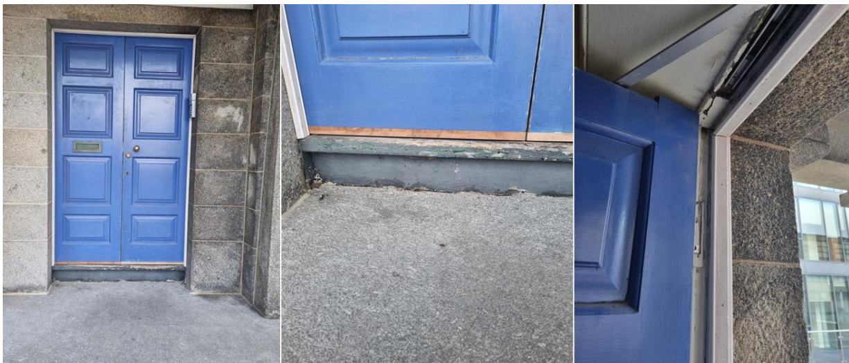
Figure 22 Slips installed on main double doors & retro seals
