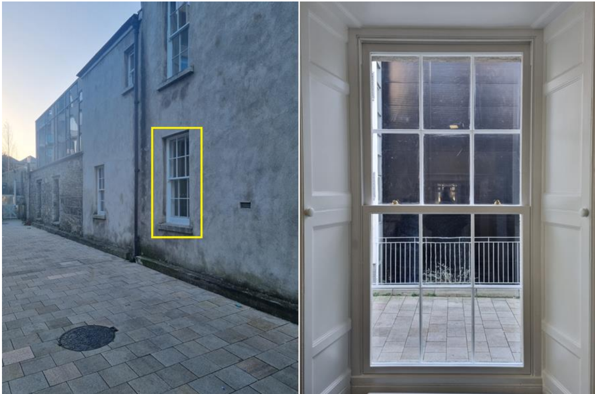
Figure 25 Blind to be installed on one window adjacent to pedestrian walkway
