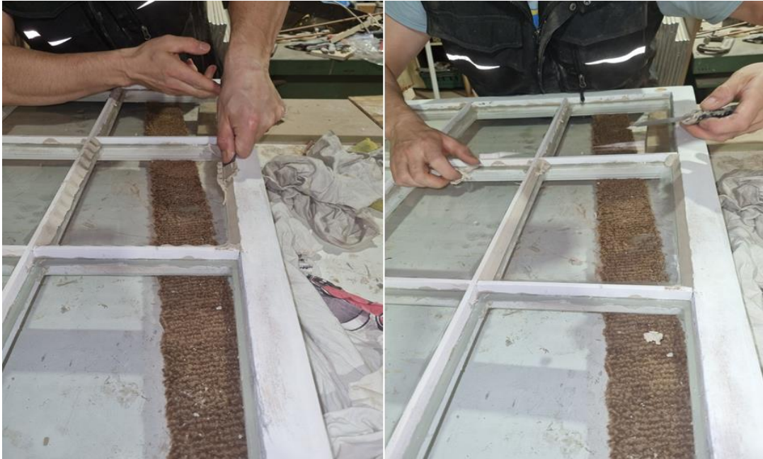
Figure 7 Glazing installed with linseed putty
