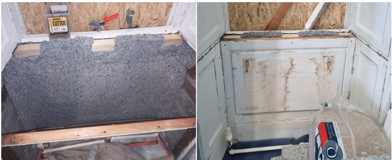
Figure 15 Boardroom window 4 east insulated with 50mm Pavacell & panel reinstalled
