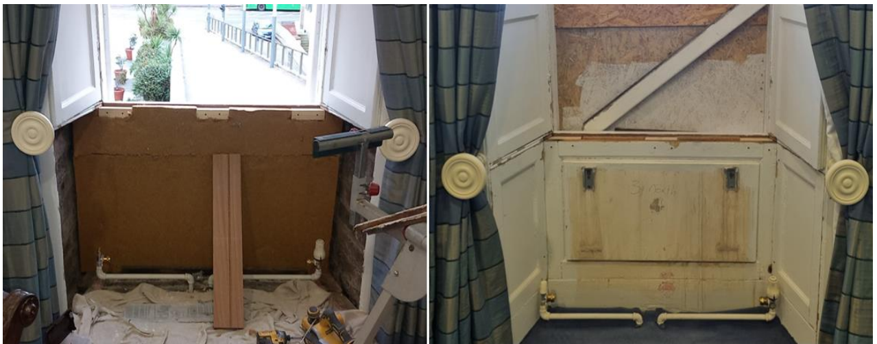
Figure 14 Boardroom window 3 north insulated with 80mm Woodfibre & panel reinstalled
