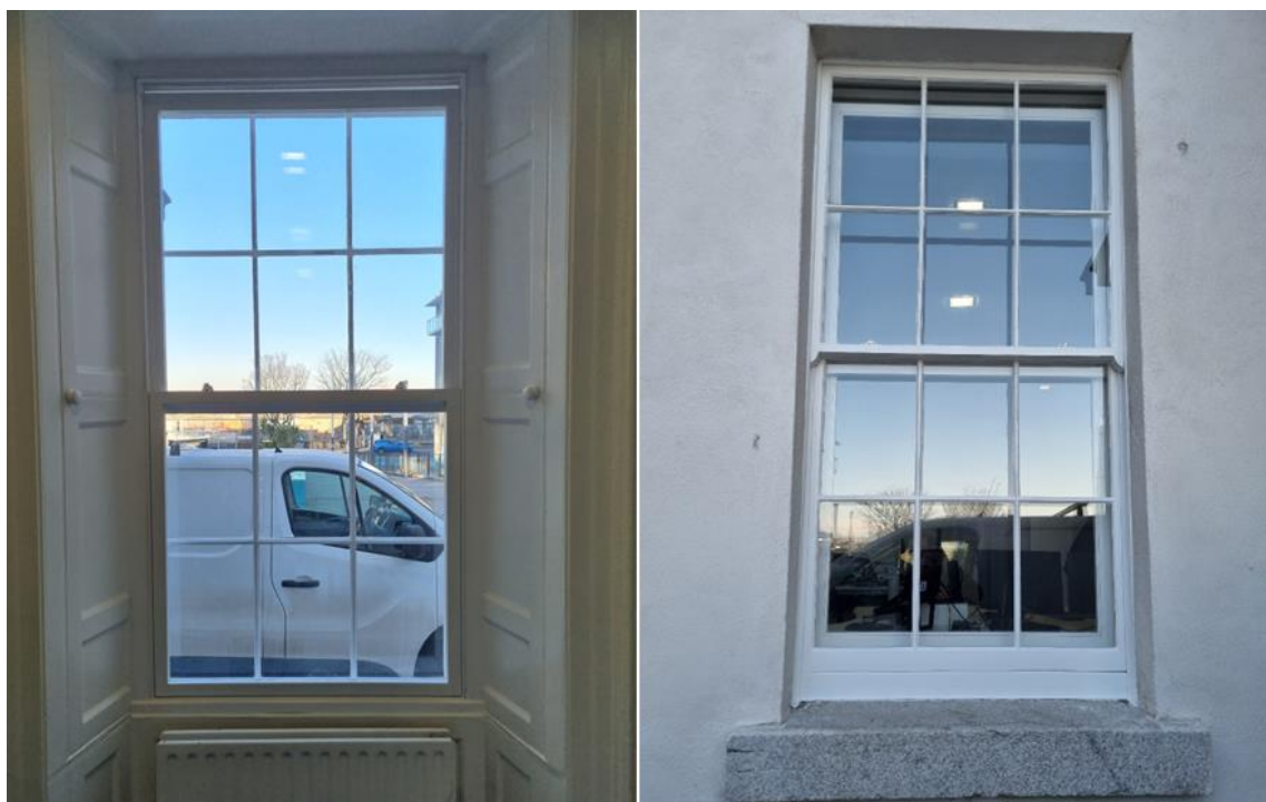
Figure 23 Inside & outside view of secondary glazing complete on ground floor office
