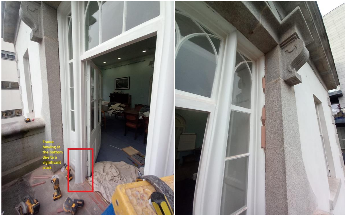
Figure 26 Areas repaired at the balcony doors
