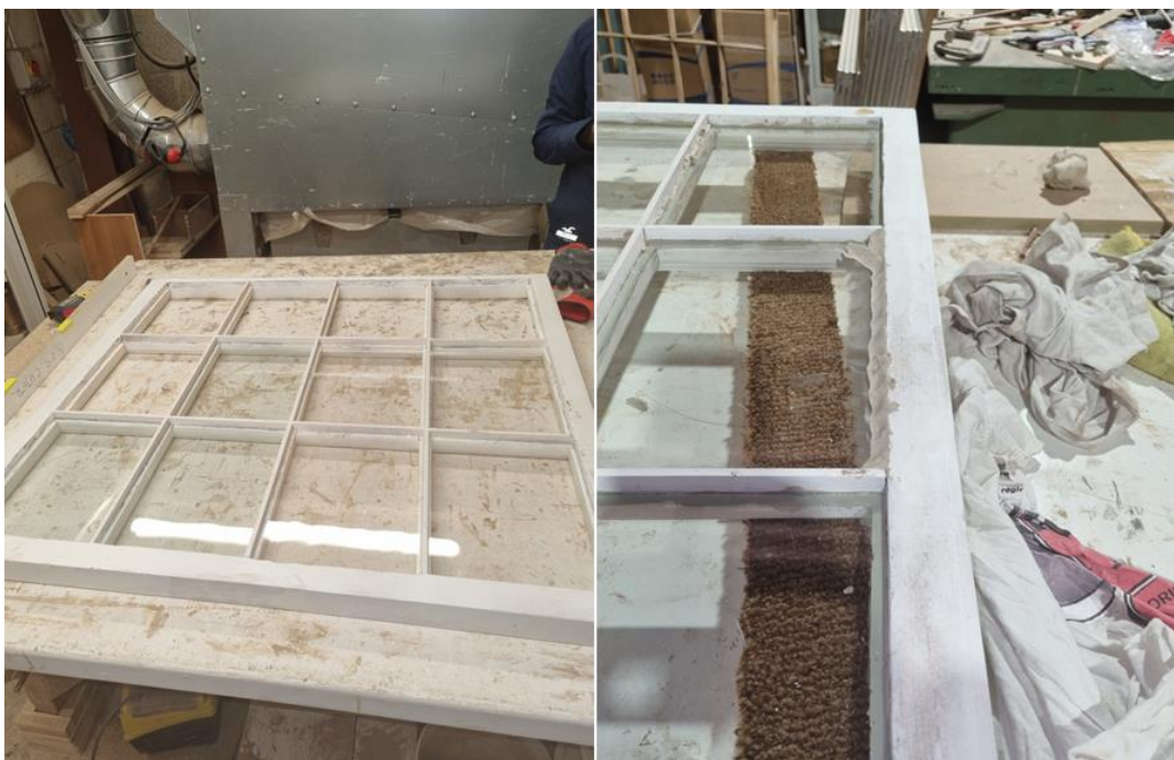
Figure 6 Frames painted & ready for glazing
