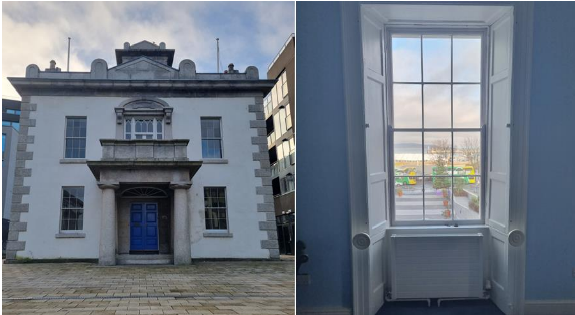
Figure 21 View of original refurbished windows - inside & out
