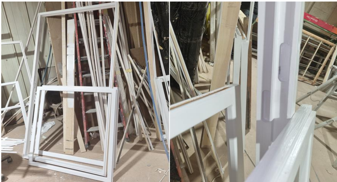
Figure 8 Secondary glazing frames - unfinished
