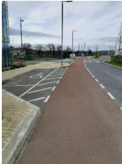
Figure D-11: Access to parking bay
